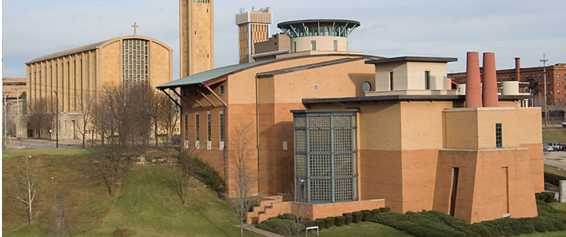
Figure 17: The Youngstown Historical Center of Industry and Labor, designed by architect Michael Graves
