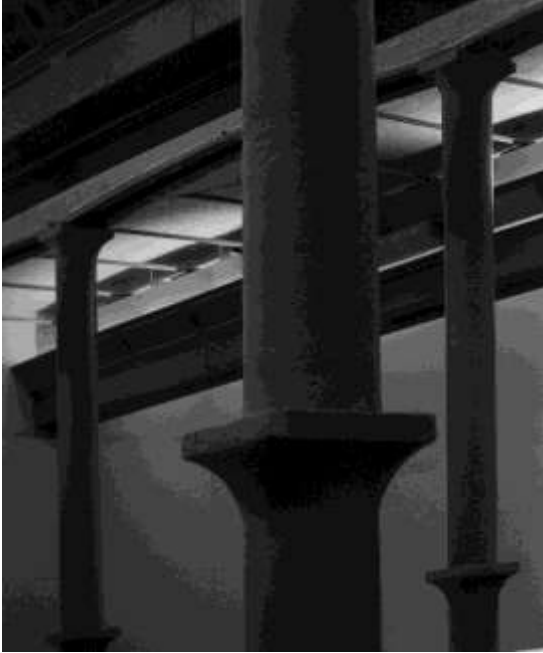
Figure 68. A column capital detail. (Tate Archive)
