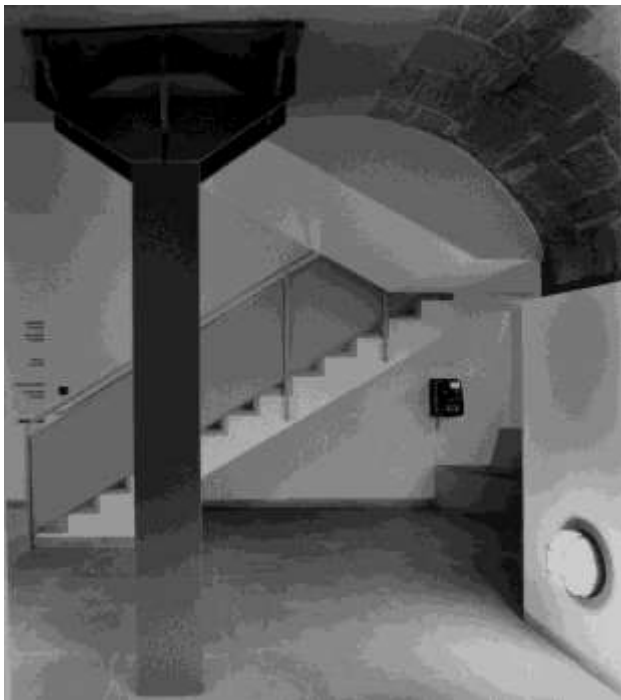
Figure 71. This view of the basement lobby clearly shows the mix of old and new materials including an exposed brick arch, steel supporting column, and white walls. (Tate Archive)
