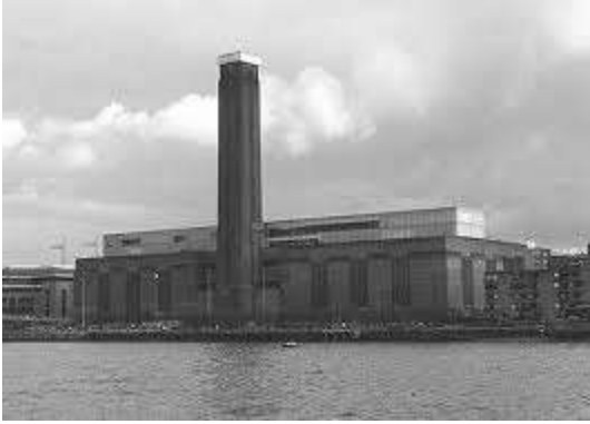
Figure 86. Tate Modern: Facade viewed from the Thames. Herzog and de Meuron's 2000 conversion retained the shell and chimney of Sir Giles Scott's Bankside Power Station. (The Tate, www.tate.org.uk )
