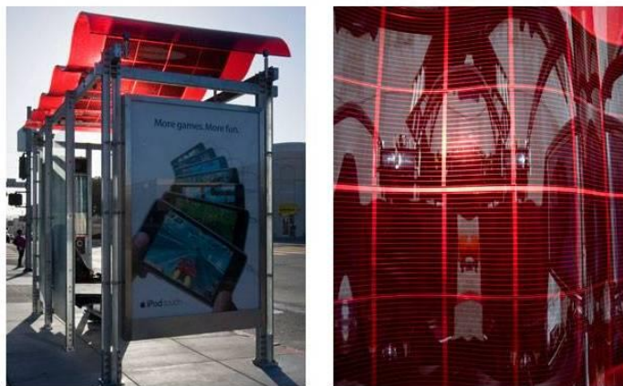
Figure 1.12 Curved OSCs installed on the bus shelters in San Francisco.
