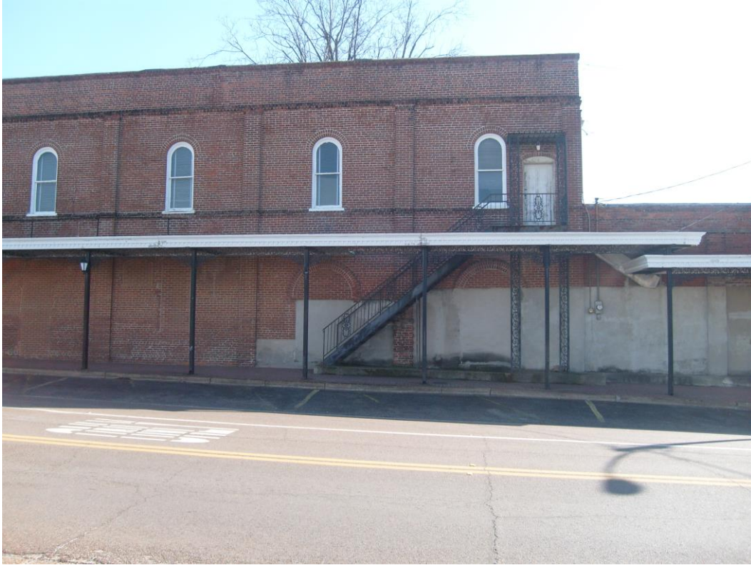
Figure 3.4: Exterior of Police Station in Cookie's Fortune as seen in 2014 (Photo taken by author).
