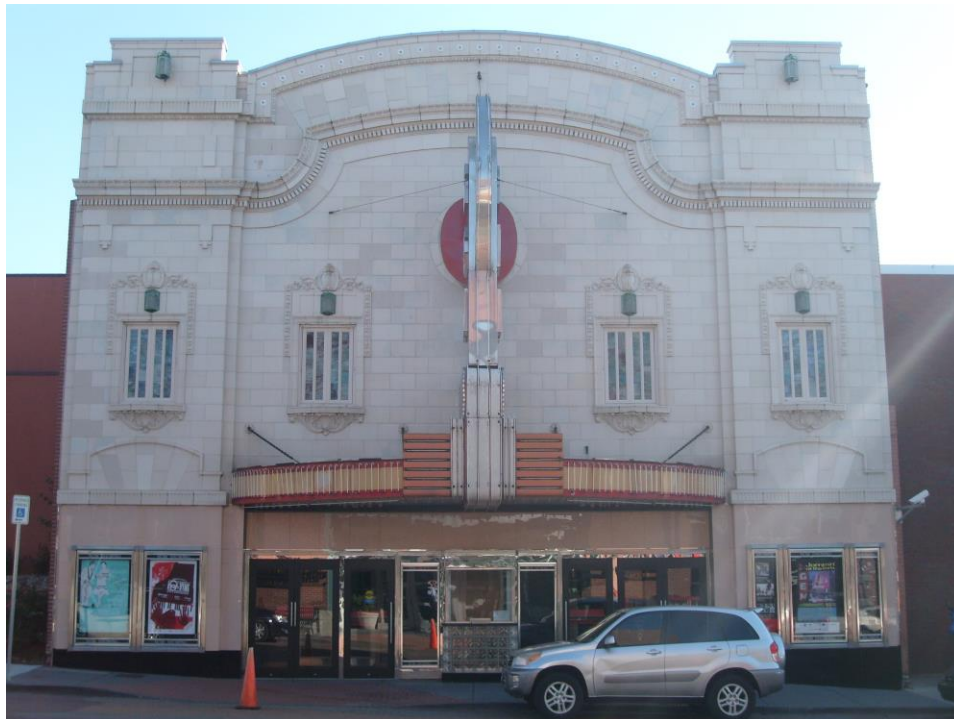
Figure 3.19: The restored historic Gem Theater, directly across the street from the Jazz Museum on 18 th Street (Photo taken by author).
