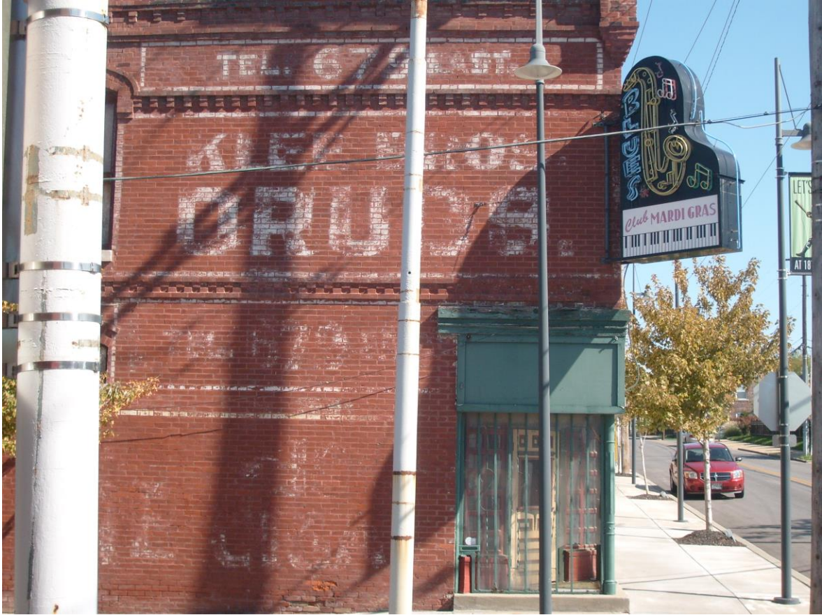
Figure 3.20: Certain production design elements remain on Vine Street almost 20 years later even though the buildings remain empty (Photo taken by author).
