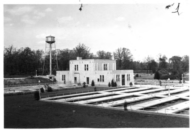
Fig.2.--City of Ann Arbor's sewage disposal plant, located along the Huron River east of Dixboro.
