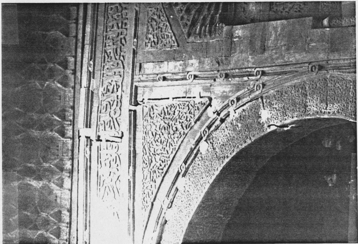
Fig. 6 Interior of El-Ghuri Mosque with plaster strips across some of the cracks
