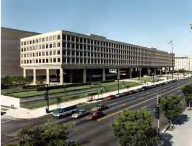
U.S. Department of Energy Headquarters
