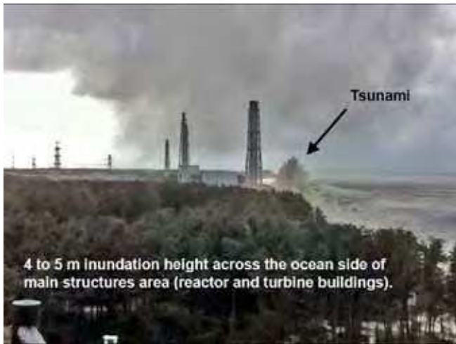
The size of the resulting tsunami was far above the seawall design of the Fukushima nuclear power station.
