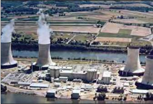
The Three Mile Island nuclear plant
