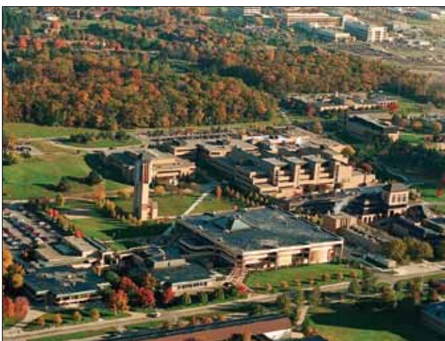
2000s The Engineering Campus is complete.
