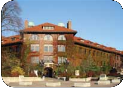
West Engineering Building
