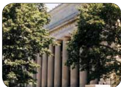
Angell Hall Renovation
