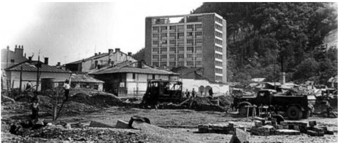
Figure 8 – View of the single's dormitories before the demolitions on Strada Mare and the reconstruction of the city center.
