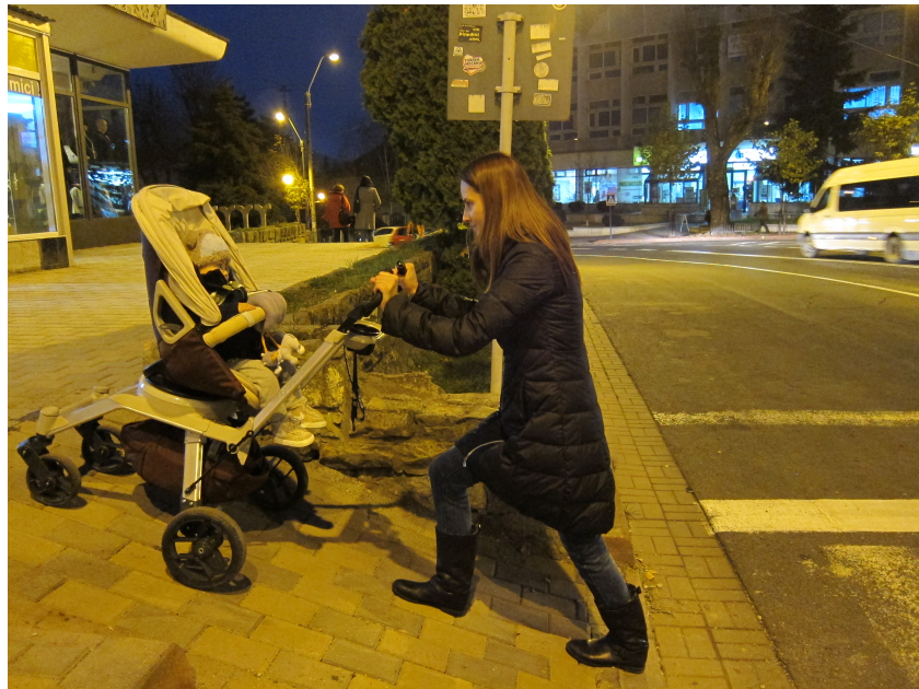
Figure 15 – Extremely steep ramp
