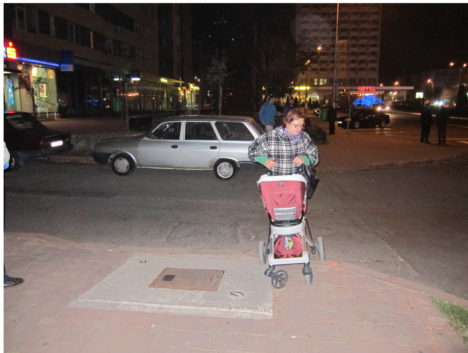
Figure 16 – Disfunctional curb ramp (photo credit Andra Lungu)
