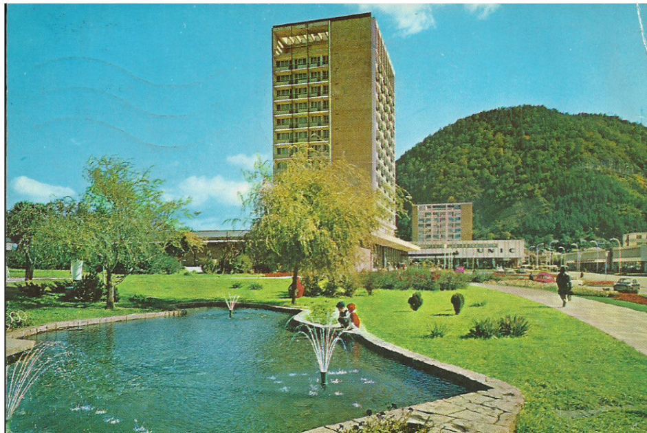
Figure 9 – View of the Ceahlau Hotel (single's dormitories in the back) from the Stefan cel Mare Park in the center
