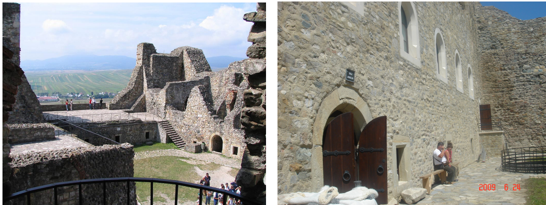
Figure 25 – left: before restoration; right: after restoration
