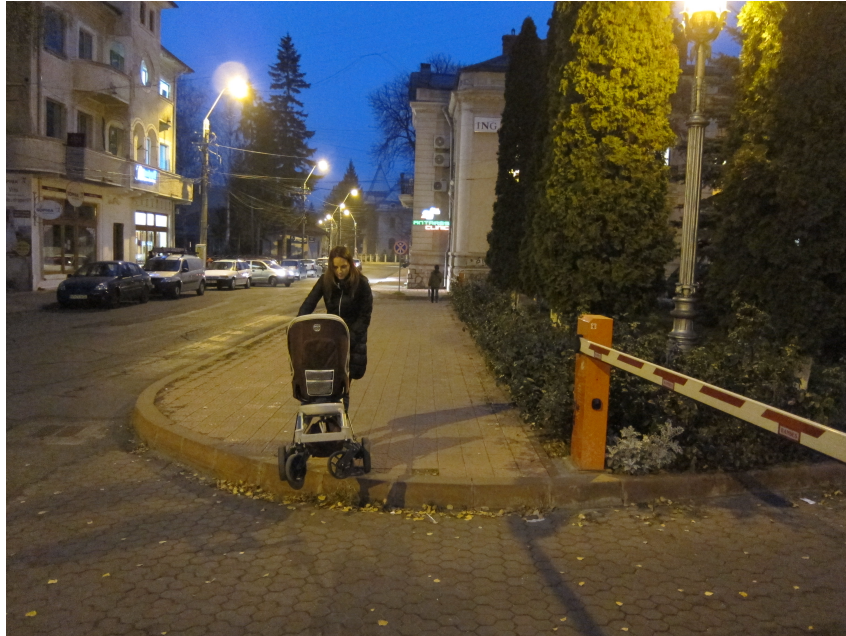
Figure 14 – New sidewalk curb with no ramp (photo credit Andra Lungu)
