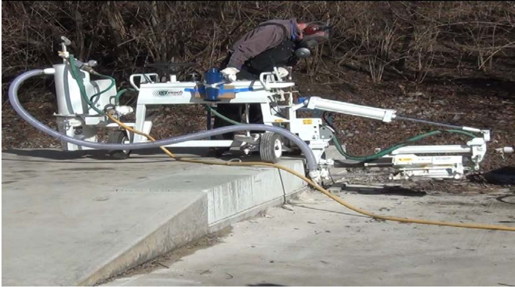
Figure 4.2 Raised concrete platform with removable concrete slabs
