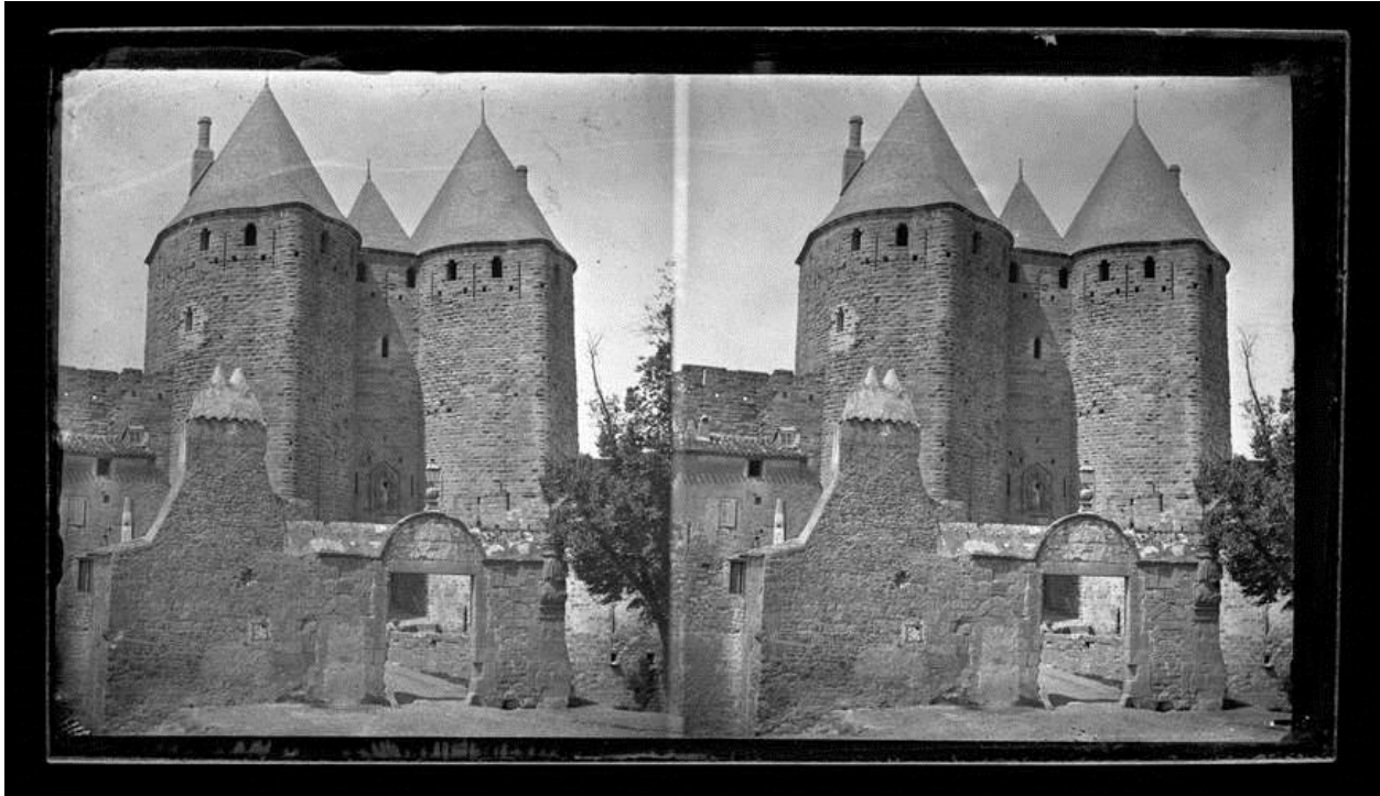
Fig. 19. The Porte Narbonnaise along the walls of Carcassonne in 1862. Photograph of Eugène Trutat. A.M.T. 51Fi178.
