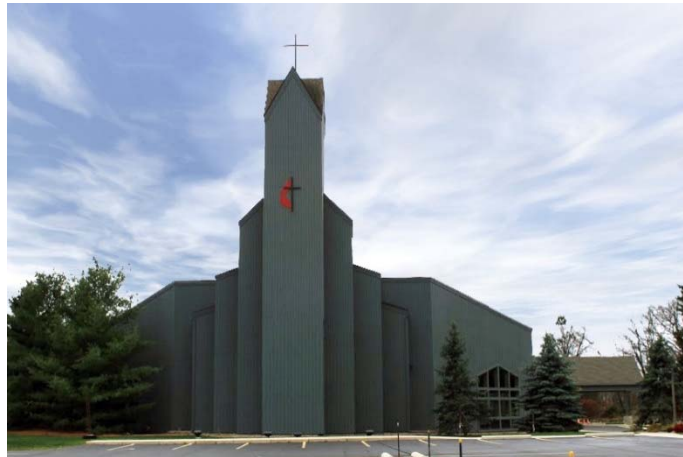
Figure IV- 6: Dexter United Methodist Church Building
