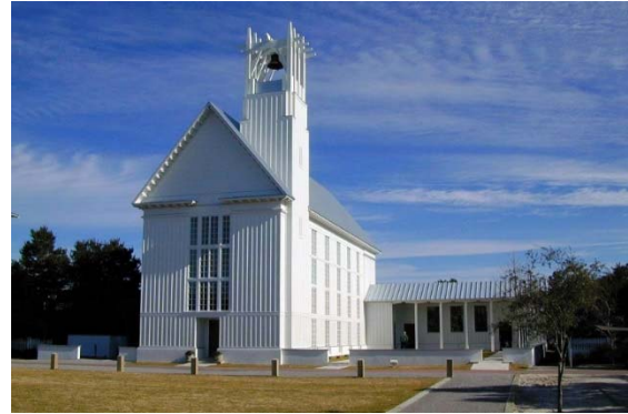
IMAGE 6 6 Seaside Chapel Seaside, Florida S, NH, R, MIX
