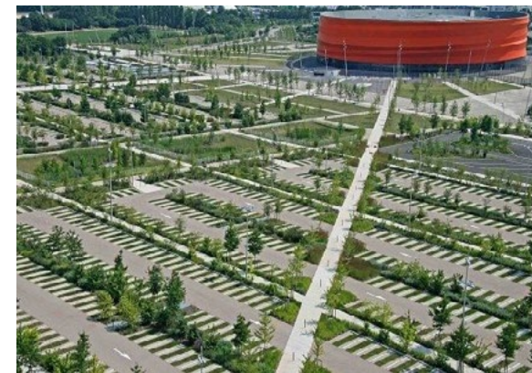
Figure - 64 Zenith de Strasbourg example of grasspave strips in parking area
