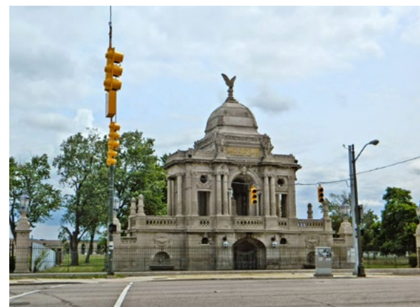
Figure - 76 View of Hurlbut Gate from Plaza
