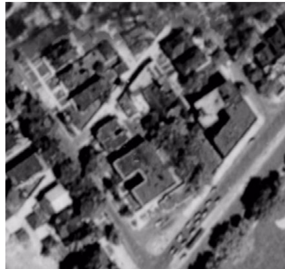
Figure - 7 Historic aerial imagery of Pewabic block (1949).
