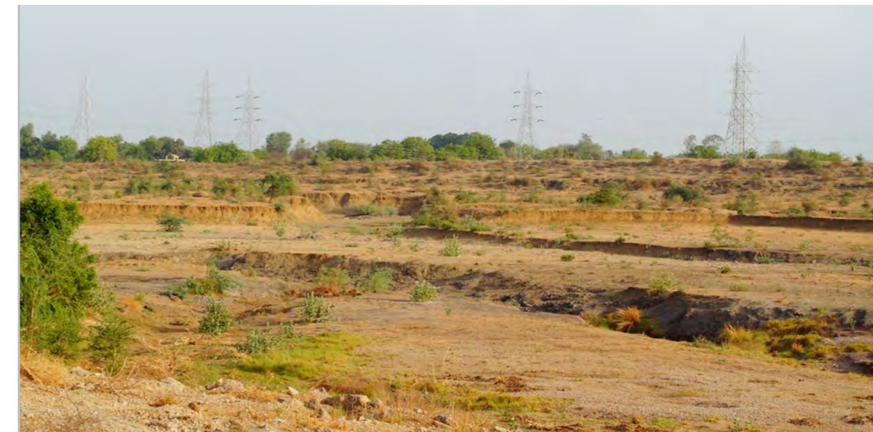
Erosion at Ajwa's outlet
