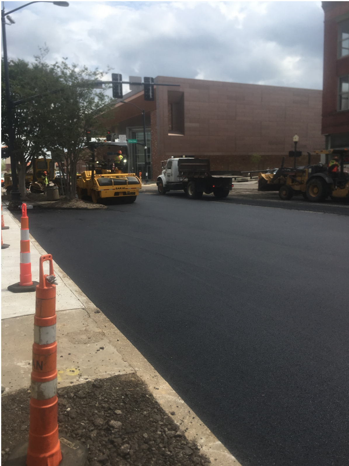
Figure 4.4e. Construction, Front Street, March/April 2018.
