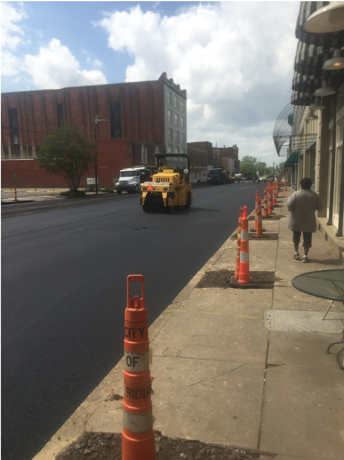
Figure 4.4d. Construction, Front Street, March/April 2018.
