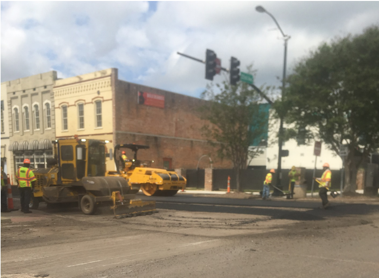
Figure 4.4a. Construction, Front Street, March/April 2018.
