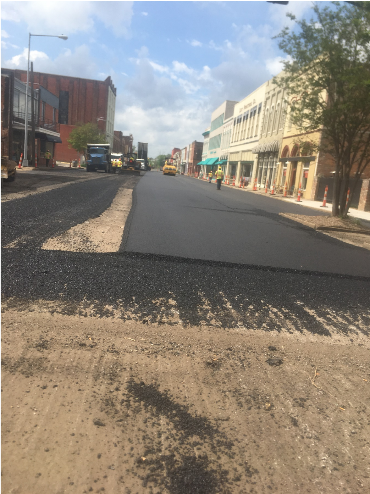
Figure 4.4c. Construction, Front Street, March/April 2018.
