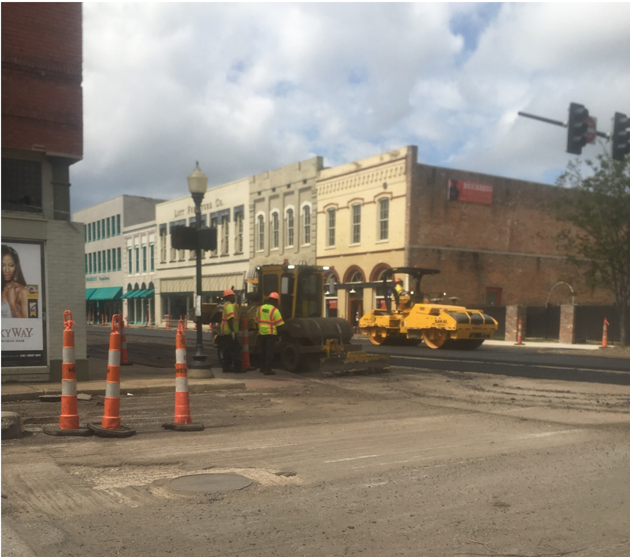
Figure 4.4b. Construction, Front Street, March/April 2018.
