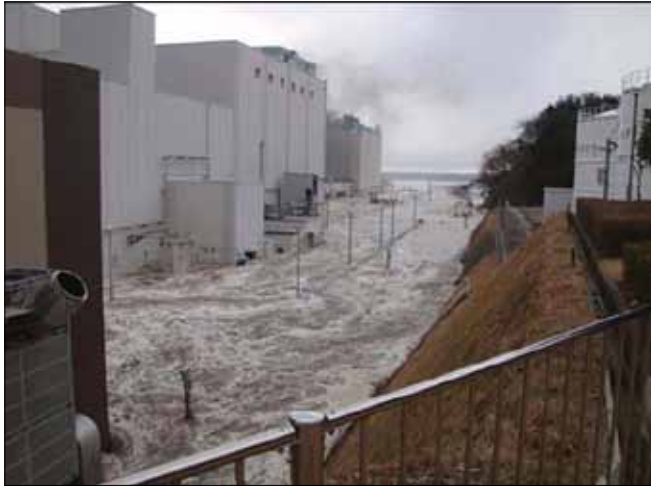
Tsunami destroys emergency cooling system
