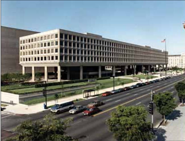
U.S. Department of Energy headquarters
