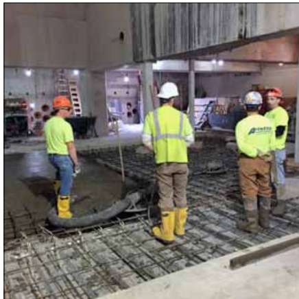
Filling the reactor pit with concrete
