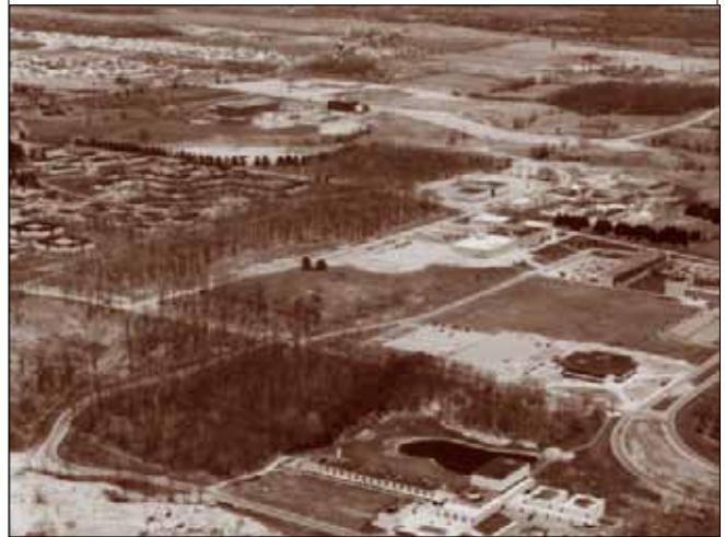
Early work on the North Campus
