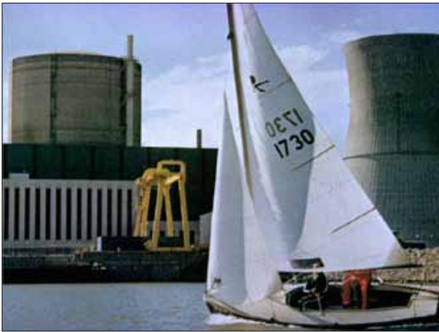
Davis Besse nuclear power plant (Ohio)
