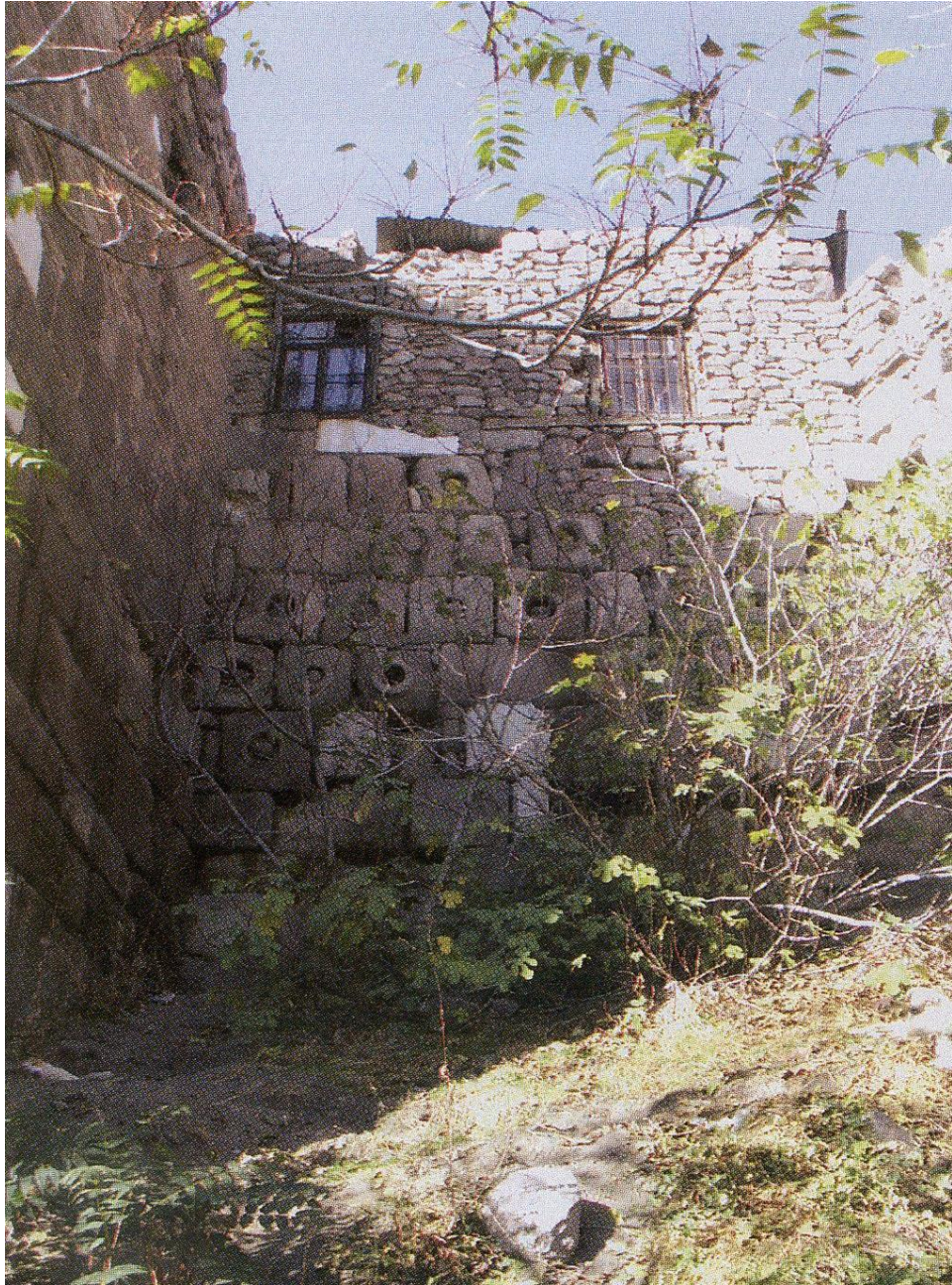
Figure 3.60. Pierced stones from the aqueduct reused in the Byzantine Citadel. (Peschlow 2015, Taf. 83, abb. 297).
