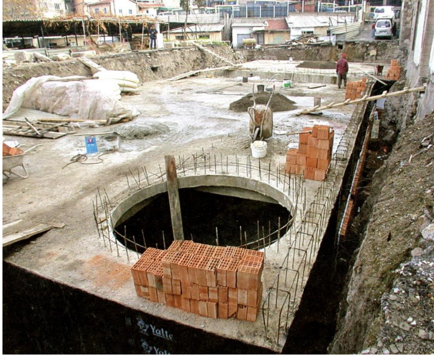
Figure 3.51. View of the boiler room. (After Kadioğlu Görkay Mitchell 2011, p. 149, fig. 80).
