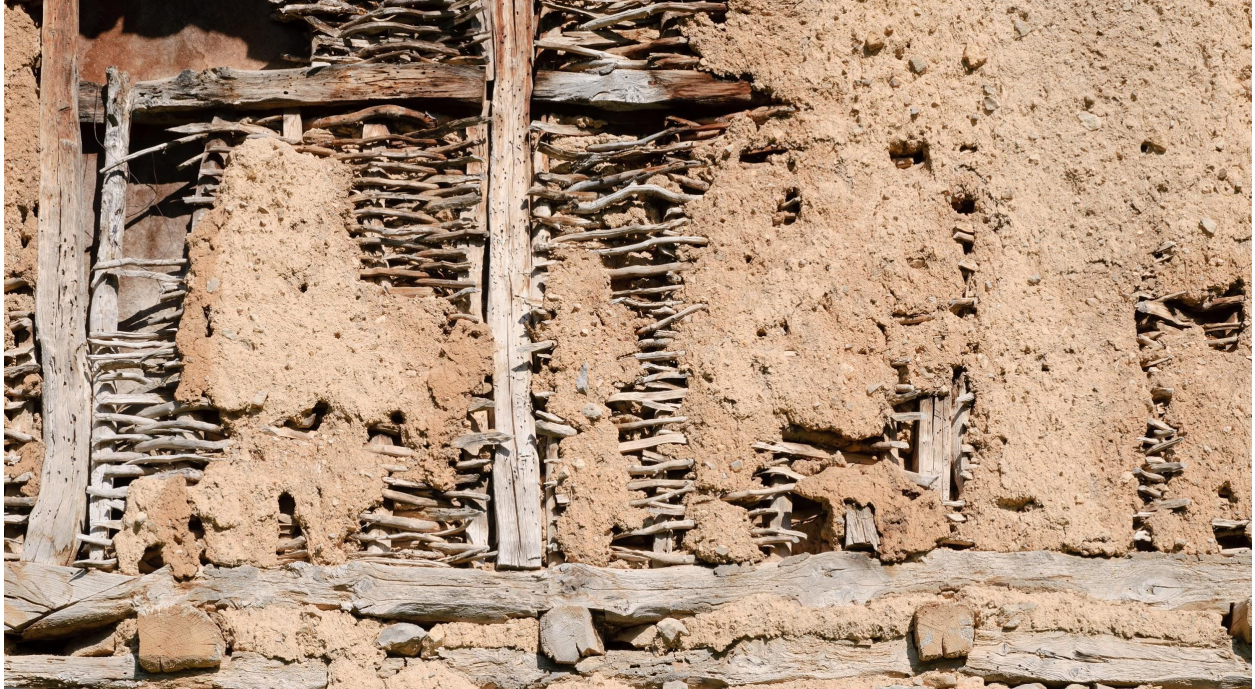
Figure 1: Example of wattle and daub construction method. Photograph by MrPanyGoff, distributed under a CC BY-SA 3.0 license at https://upload.wikimedia.org/wikipedia/commons/e/e5/Wattle_and_daub_construction.jpg
