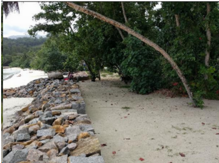
Figure 3.3: Rock Armoring found along Anse A La Mouche. (Reguero et al. 2018)
