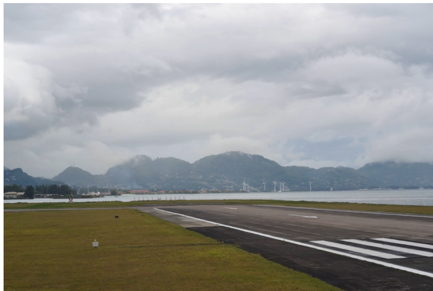
Figure 2.3: Runway at Seychelles International Airport at Mahé
