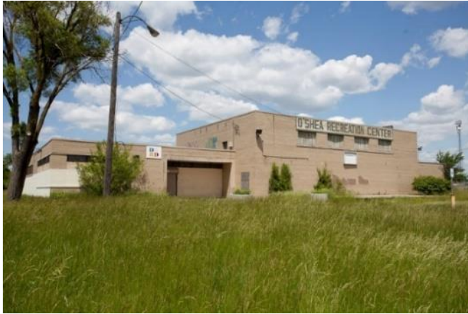
Figure 19: O'Shea Recreation Center, pre-demolition (DetroitUrbex.com, 2018)
