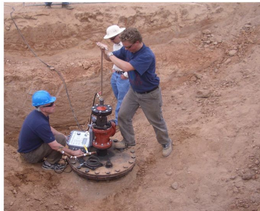
Figure 1. Inserting an Acoustic Device to Detect Leaks in a Pipe Line [1]
