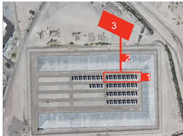
Figure 7. The Palo Verde Generation Station in Tonopah, AZ site used for dependent variables in our mathematical model. The red annotations indicate our physical solution on site, highlighting the (1) dry storage casks, (2) duct-fan system for heat transport, and (3) application area.
