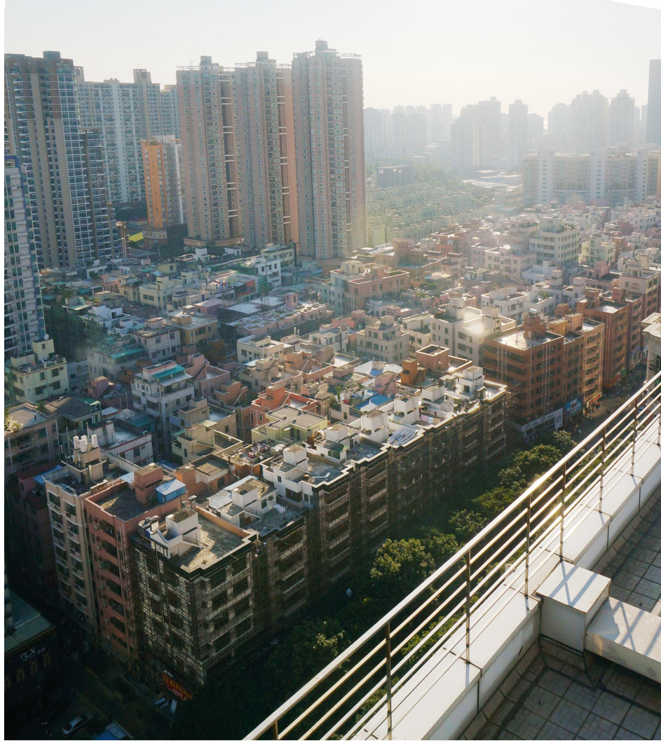
Figure 2-13. An aerial view of Shuiwei Village in the Futian District, Shenzhen 2016
