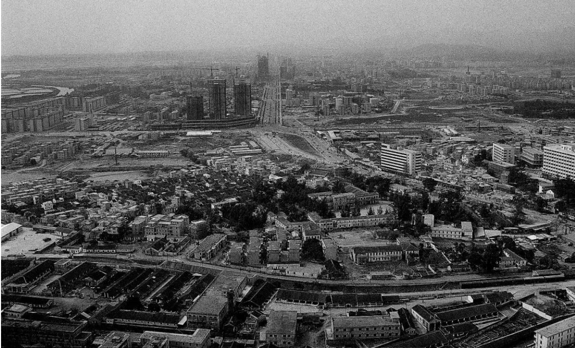
Figure 3-9. Urban structures built around the Caiwuwei Village in 1985
