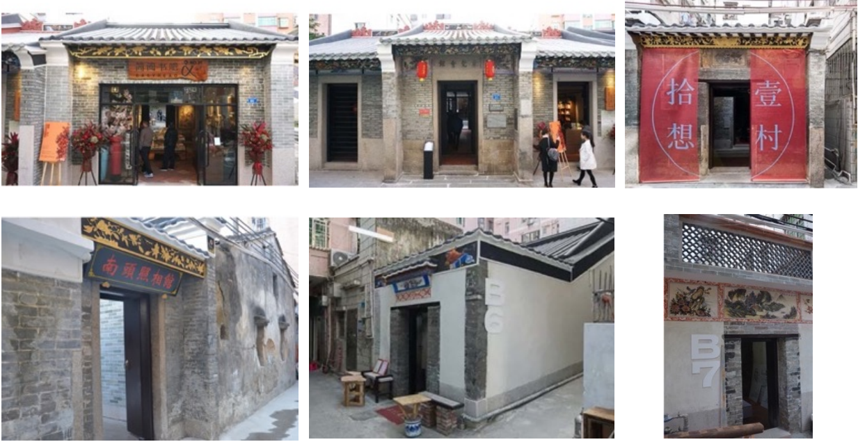
Figure 5-3. Six renovation projects of old courtyard houses at Nantou
