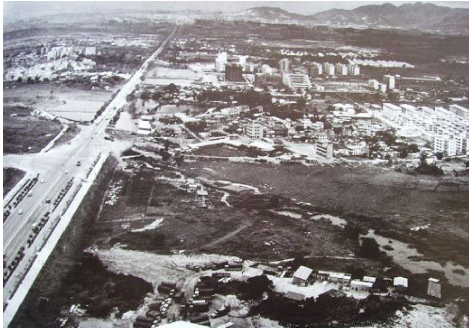
Figure 2-24. An aerial view of the Shennan Avenue under construction in 1982
