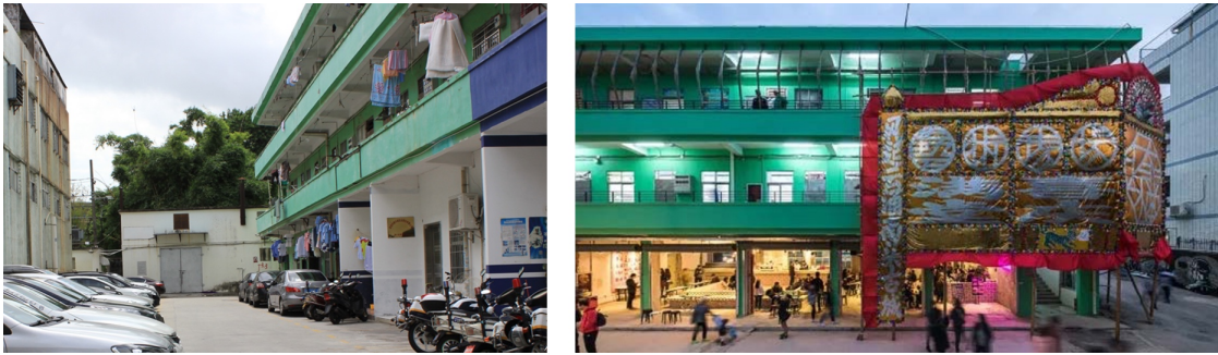
Figure 4-13. Left , a worker's dormitory located at the old factory zone; right , a café on the ground floor and small exhibition rooms on upper floors
