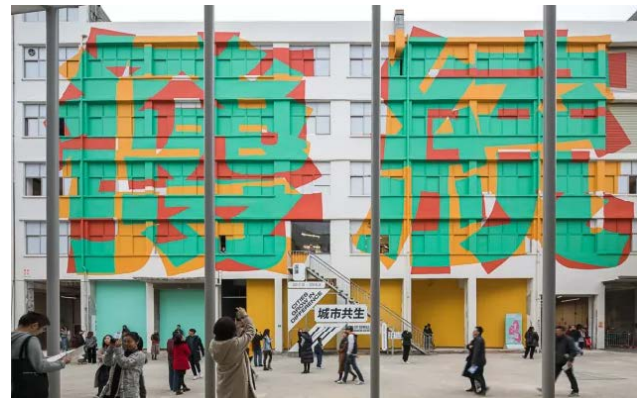
Figure 6-13. A mural on a factory building that was converted to an indoor exhibition hall
