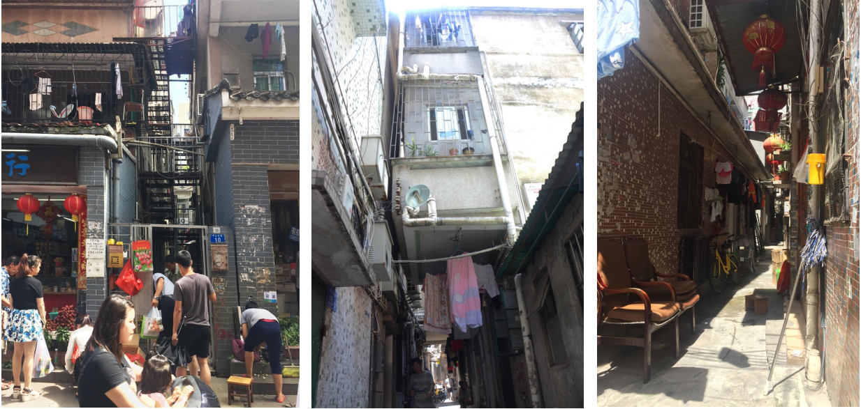
Figure 5-7. Handshake buildings at Nantou
