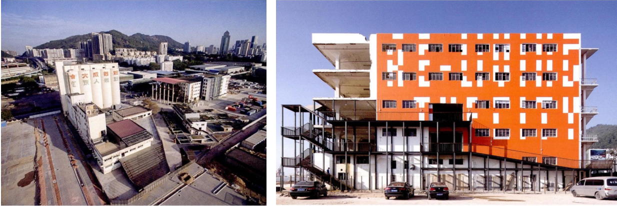
Figure 4-8. Left , the Dachan Flour Mill site at the Shekou District, Shenzhen; right , façade of the renovated No. 8 Building (Photos from Liu Heng, “Re-Living the City: The Overview of 2015 Shenzhen/Hong Kong UABB, Shekou Dachan Flour Mill, Shenzhen,” Time + Architecture 1 (2016), Fig. 3, Fig. 15)
