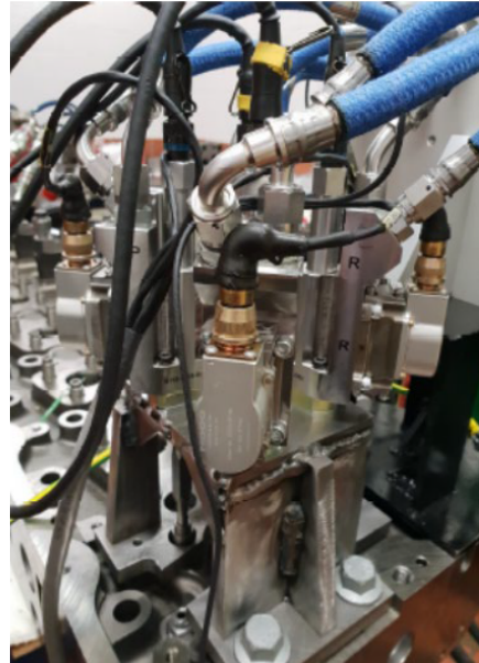
(b) Actuator base installed
