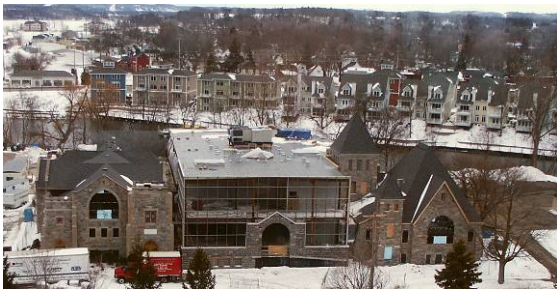
Fig 61: 2006 Courthouse expansion encompassing two stone churches with new modern structure built between them
