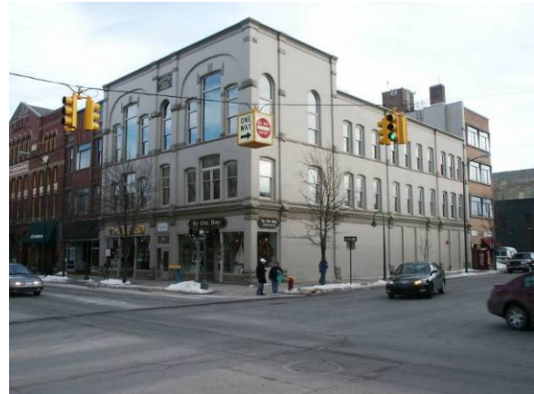
Fig 79b: The reconstructed building in 2006
