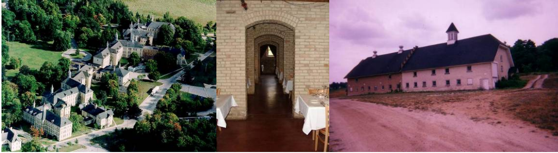
Figs 60a,b,c: Building 50 of the Traverse City State Hospital in the 1990s, Dining spaces in a restaurant in the Village at Grand Traverse Commons, Old State Hospital barn
