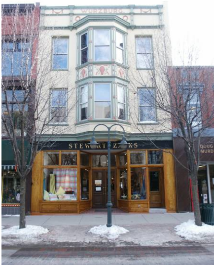
Fig 83: The Wurzburg Building in 2006
