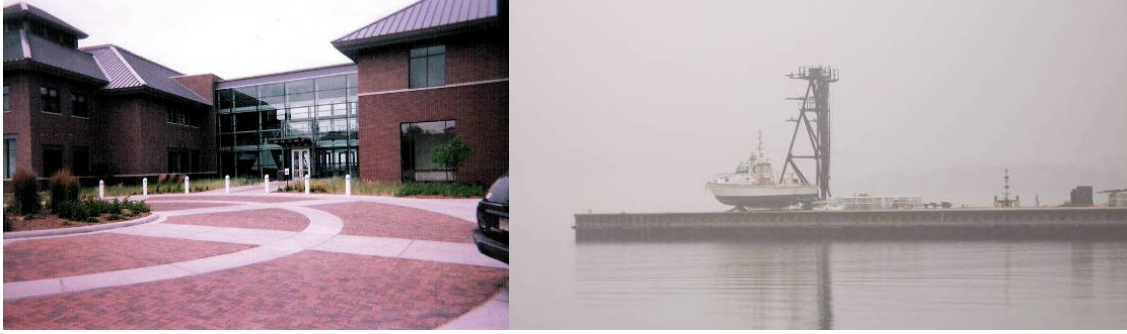
Figs 58a,b: The Hagerty Center at the Great Lakes Campus of Northwestern Michigan College, The Maritime Institute Dock
