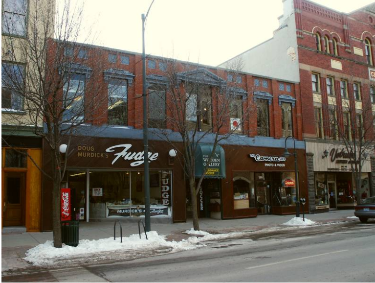
Fig 82: The Anderson Building in 2006
