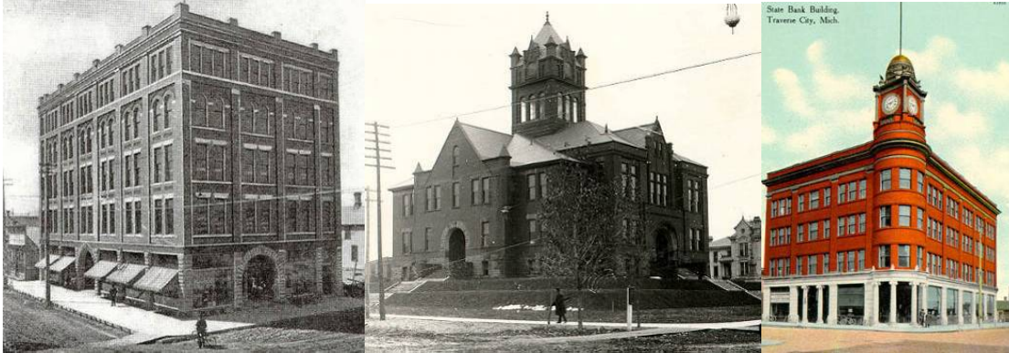
Figs 32a,b,c: The Emanuel Wilhelm building (on the southwest corner of Front and Union Streets), built 1900, The County Courthouse (on the southeast corner of Washington Street and Boardman Avenue) built 1900, The Traverse City State Bank (on the northwest corner of Front and Union Streets) built 1902
