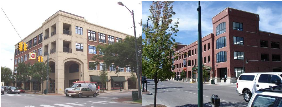
Figs 59c,d: Radio Centre (300 E. Front Street) built 2001, Larry C. Hardy Parking Deck on State St, built 2001.
