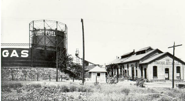
Fig 91a: Traverse City Gas Company
