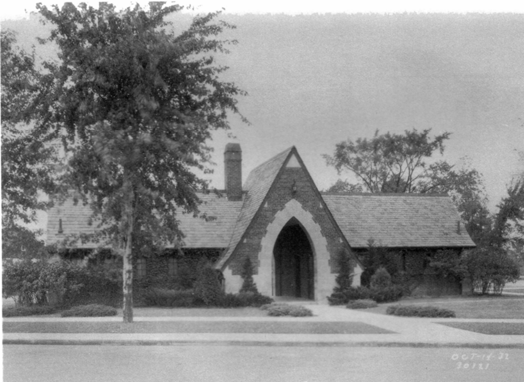
Figure 6: A comfort station in Wayne County intended to provide necessary services to motorists and park users 27
