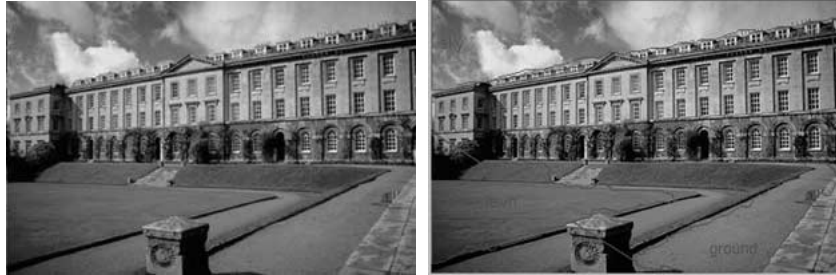
Figure 18. An example of ground and its annotation. The building is annotated with “bldg.”
