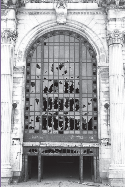
Dilapidated Detroit Train Station (photo: Patrick J. Duggan)
