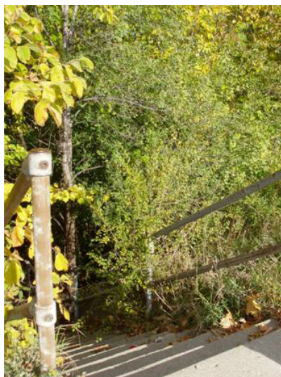
Figure 7.10: The stairway from Court Street to Aldrich Park is not very inviting.
