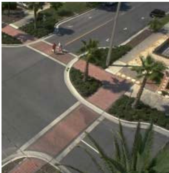
Figure 6.6: Bumpouts can be used to calm traffic and highlight parking lanes while leaving space for bicycle traffic.
