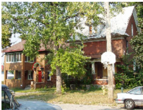
Figure 2.10: Houses in the Grand Traverse neighborhood are in varying states of repair.
