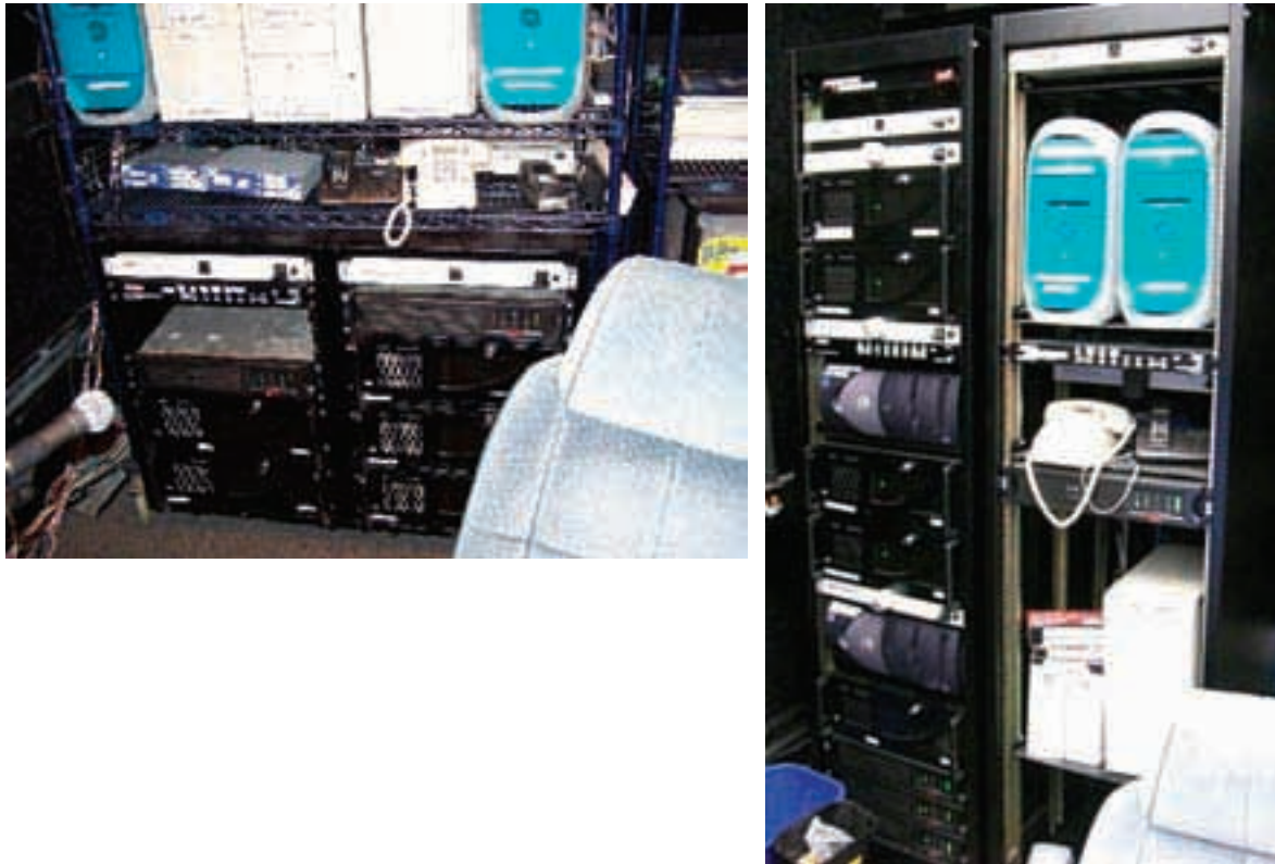
Figure 46. Before (left) and after (right) pictures of simulator racks.
