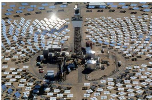
In central receiver systems (right, photo source: NREL), multiple heliostats<sup>101</sup> track the sun and concentrate solar energy into a receiver on top of a tower. Here the heat is used to produce high-temperature steam, which drives turbines to generate electricity. Central receiver systems have a solar concentration ratio of as much as 1,500.<sup>102</sup>
