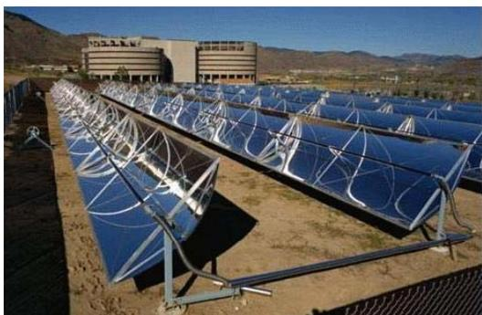
Parabolic trough systems have been around since the 1980s (first plants built in the United States), and have undergone significant technology improvements since then. However, their solar-to-electric conversion efficiencies still remain low (exacerbated by parasitic losses that can be as high as 15%), and the plants require significant stretches of flat, open land spaces. Moreover, the plants consume significant amounts of cooling water (unless dry-cooling methods are employed).
