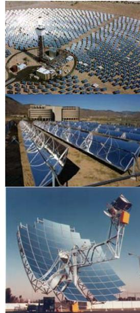
**Solar tower (top), parabolic trough (middle), dish-Stirling (bottom)**
