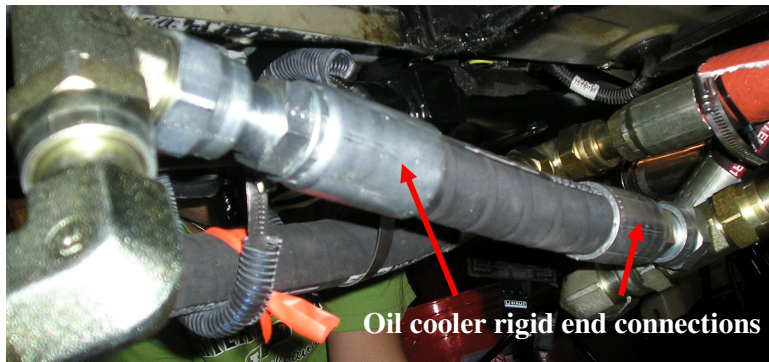
Figure 9: Oil cooler line
