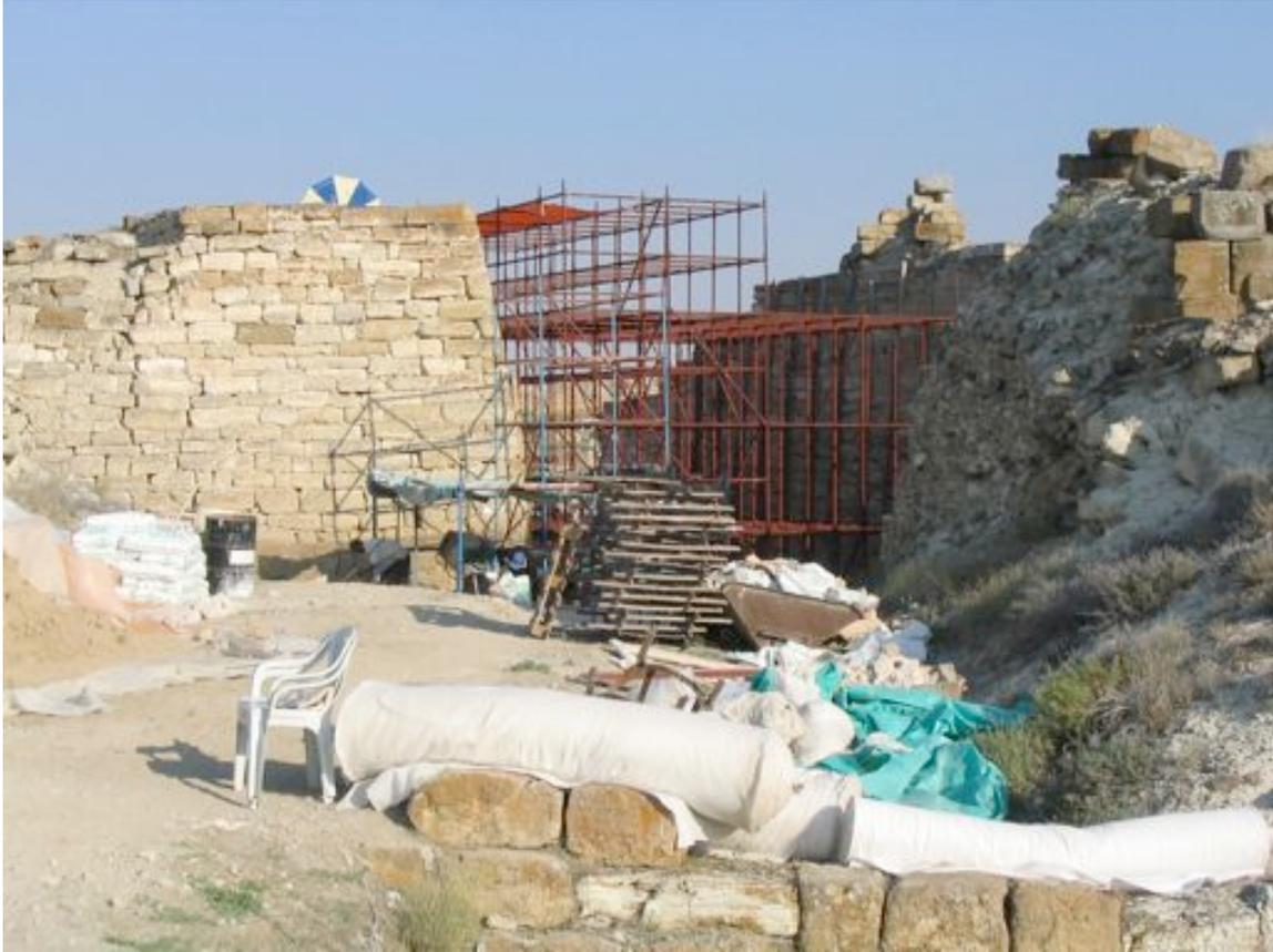
**Figure 7-4. The citadel gate, Gordion. Scaffolding allows injection of hydraulic lime into the structure (D. Shoup)**
