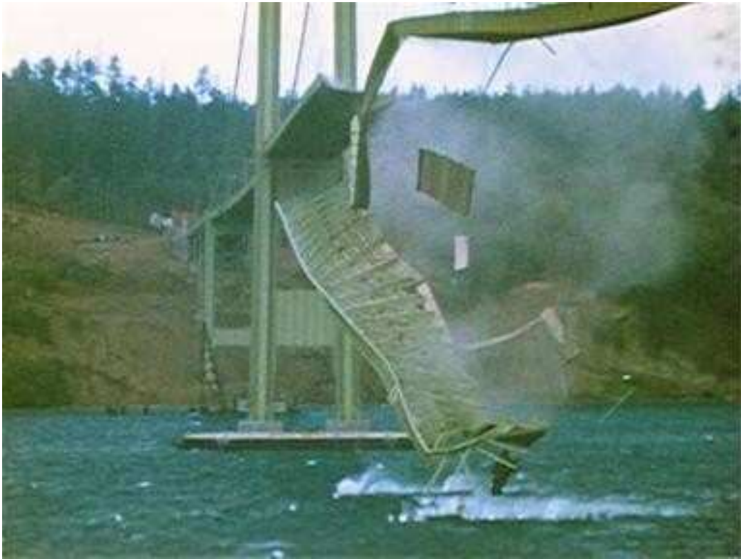
Figure 1.5: The destructive nature of VIV is best exemplified by the Tacoma Narrows Bridge Disaster in Tacoma, Washington, 1940.
