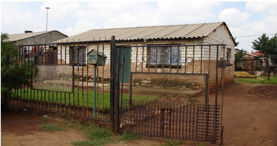
Figure 1-4: Sowetan “Matchbox” House 19
