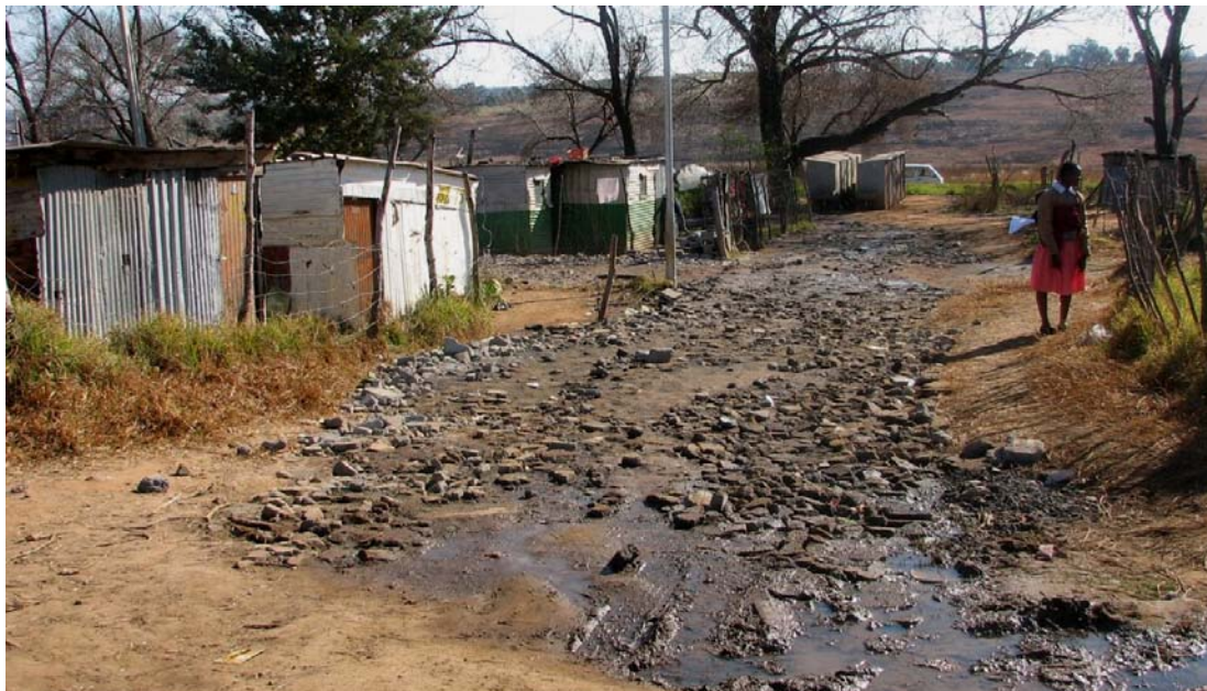
Figure 4-9: Leaking sewerage in Sol Plaatje
