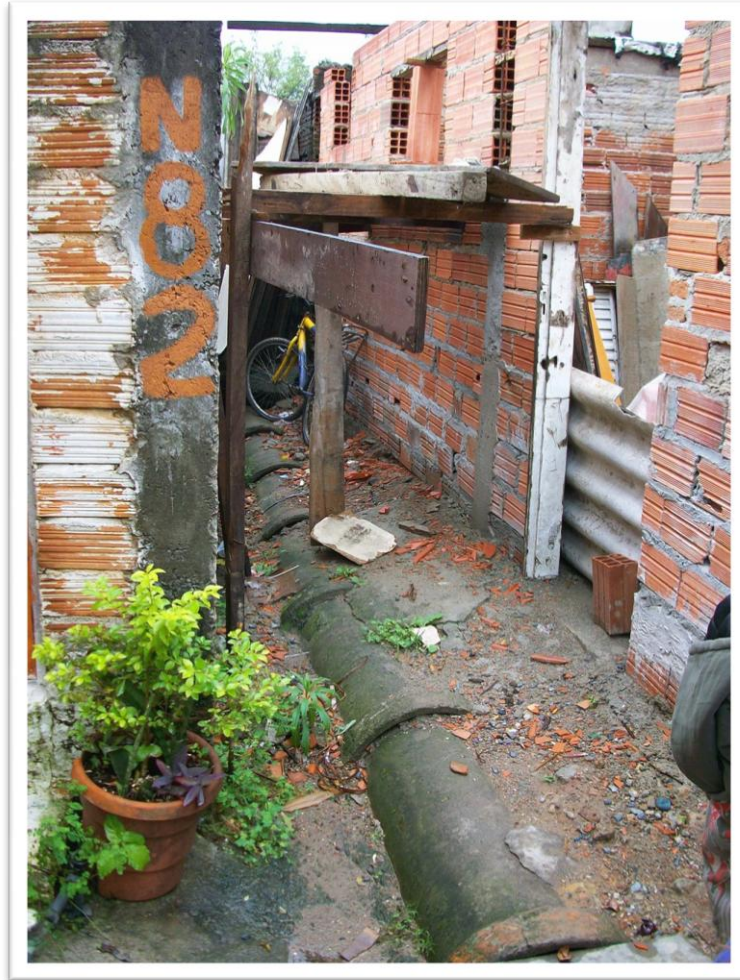
Image 10: New section of sewer line in the Santa Isabela favela. (Photo: Wilson)
