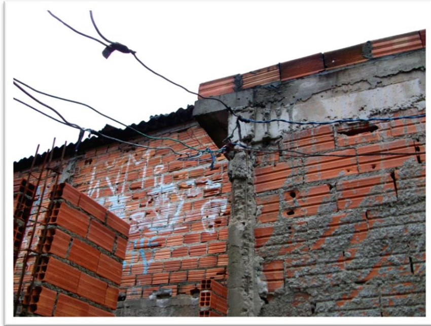
Image 11: A typical electrical connection in Santa Isabela. (Photo: Barber)
