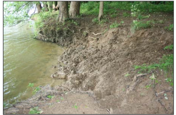
Figure 16: Erosion along the stream channel near the Westwood House
