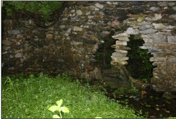
Figure 23: Historic Cool Spring infrastructure
