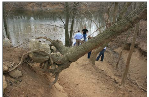
Figure 17: The shoreline east of Westwood House is badly eroded and needs restoration and stabilization
