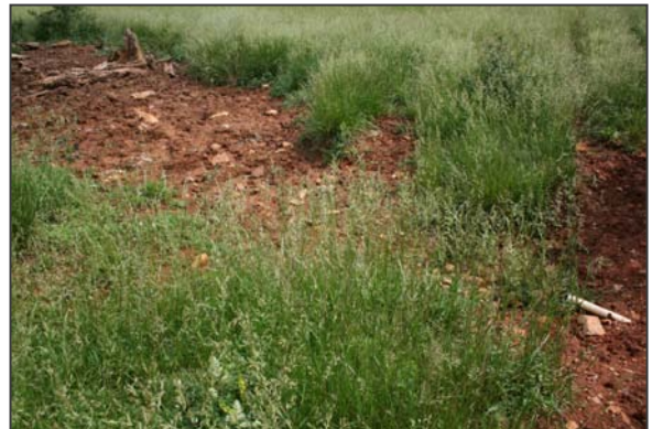
Figure 21: Storm drain pipe (lower right) causing mud and erosion behind the Retreat House
