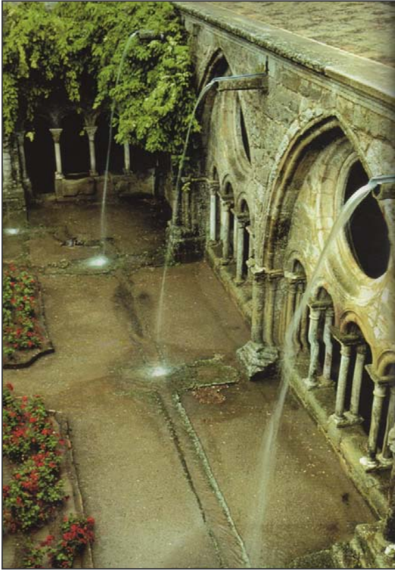
Figure 28: A historic Cistercian approach to drainage at Fontfroide Abbey in Franc (it would be better if these gutters emptied into a vegetated area)
