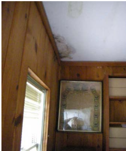
Figure 15: Mold in small office space adjacent to St. Joseph's Scriptorium
