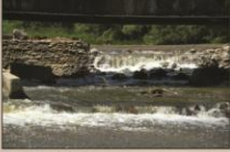
Partial removal of Mill Creek Dam in 2008
