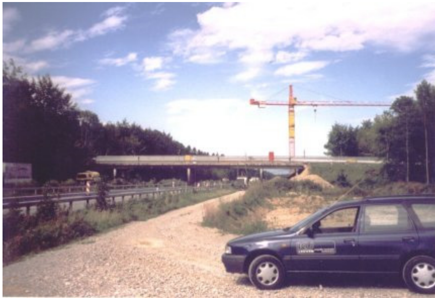
Figure 5.4. Z24 bridge (Photo courtesy of Verbraken (1999)).
