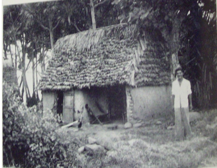
Figure 2.9 Sugar cane thatched house with earth walls in northeastern lowlands
