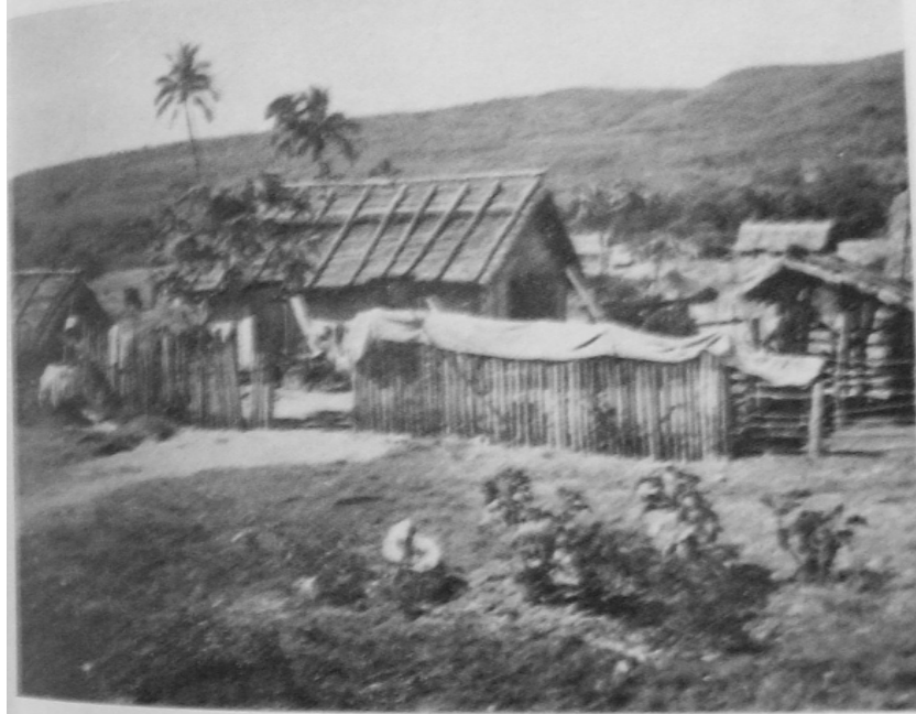
Figure 2.8 Thatched house with woven calumet walls on the west coast
