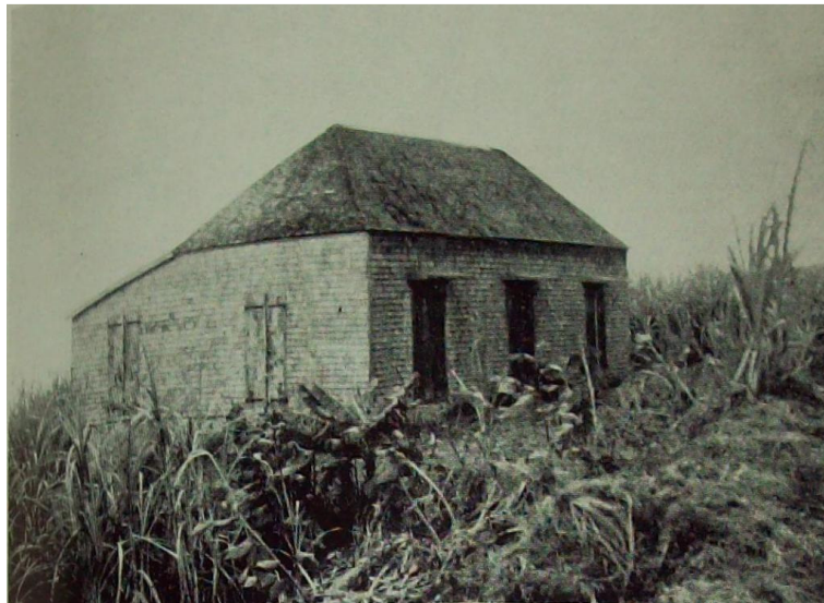
Figure 2.11 Small landowner's house, Etang Salé les Hauts
