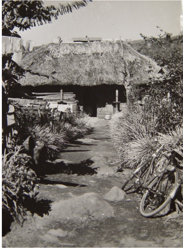
Figure 2.10 Thatched house with wood plank walls and kader garden barrier
