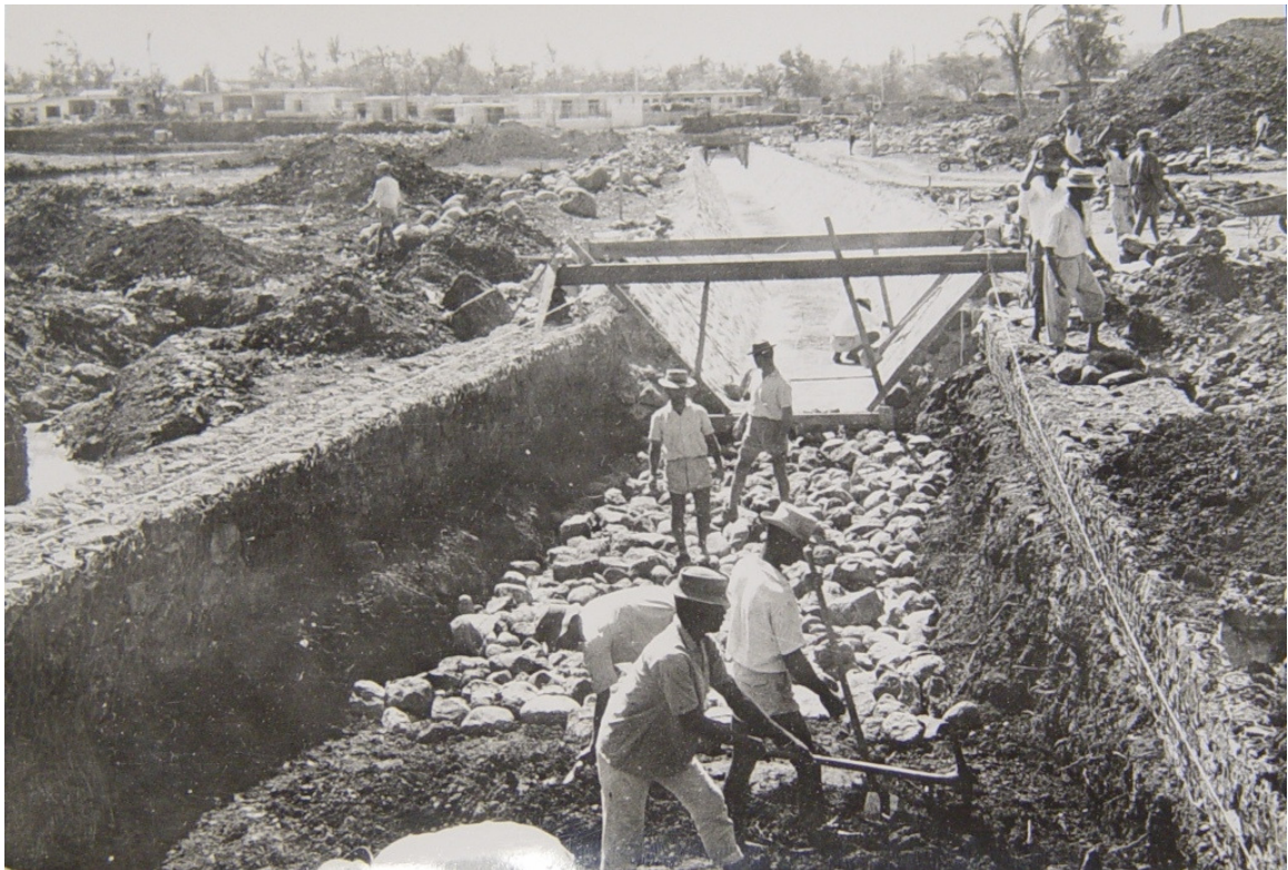
Figure 3.4 Construction workers in St Denis c1961
