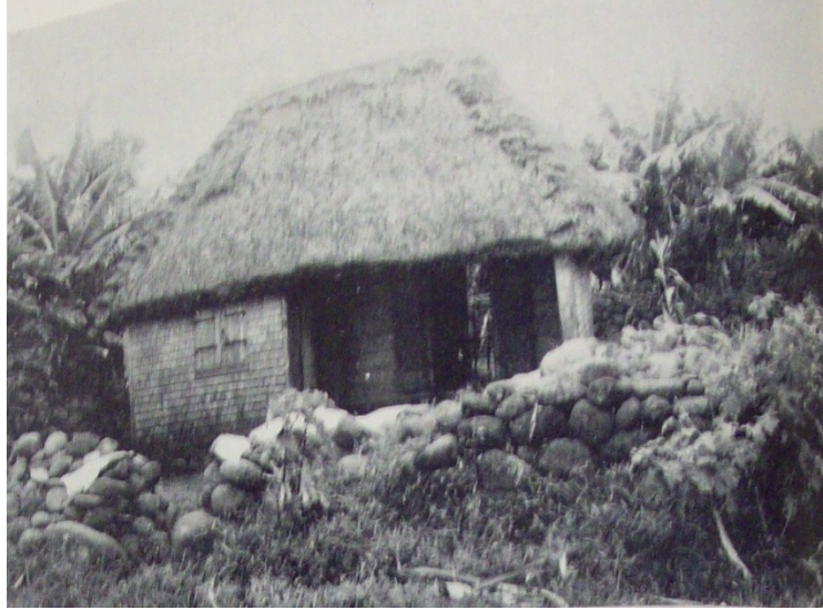
Figure 2.6 Thatched house with wood shingle walls in northeastern lowlands
