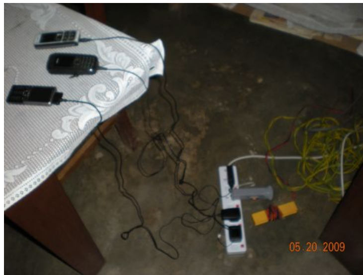
Figure E.5: Appliances at a cellphone charging station
