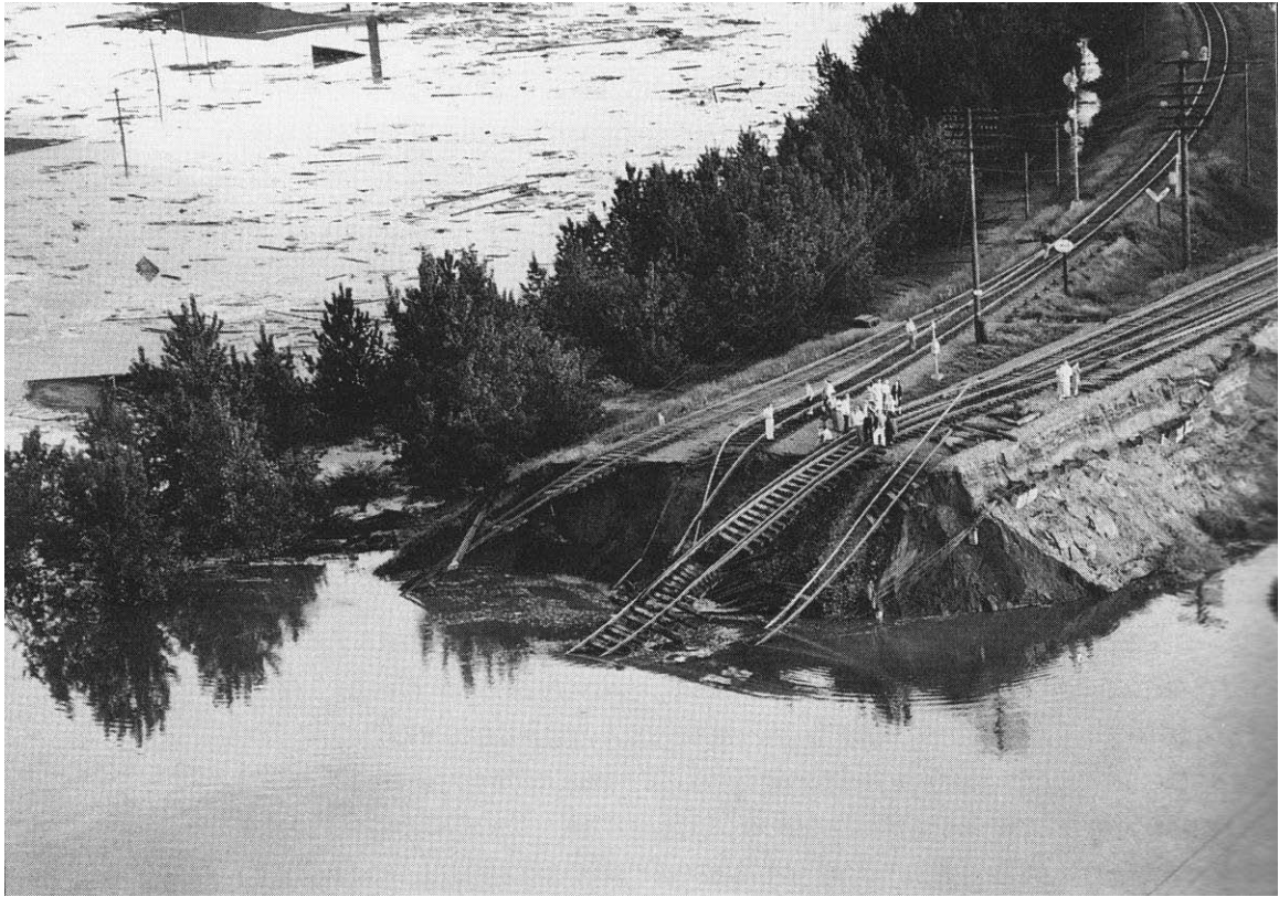
Breach in the Railroad Dike. 1948. The source of the inundation, the failed railroad dike was 125 feet wide at its base and 75 wide at its top.
