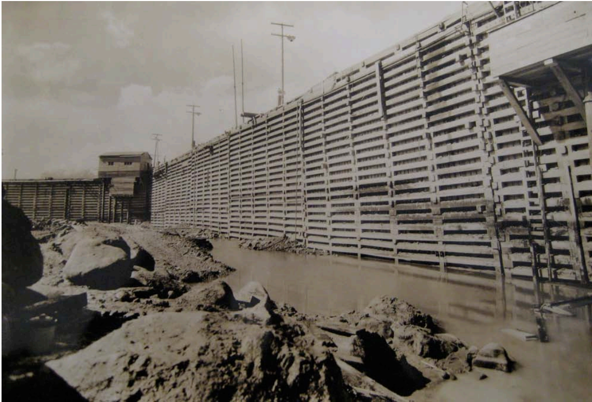
Inside the Cofferdam.
