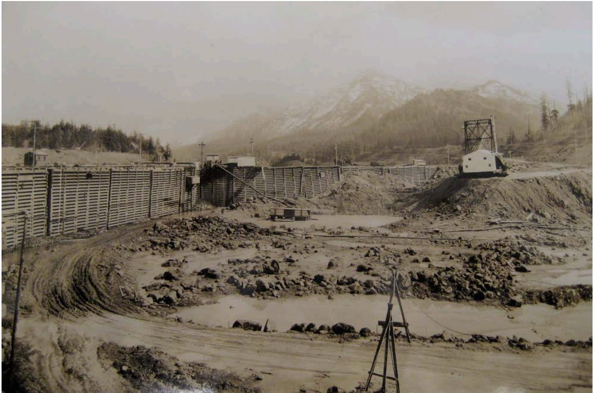
Inside the Cofferdam, Wide View.
