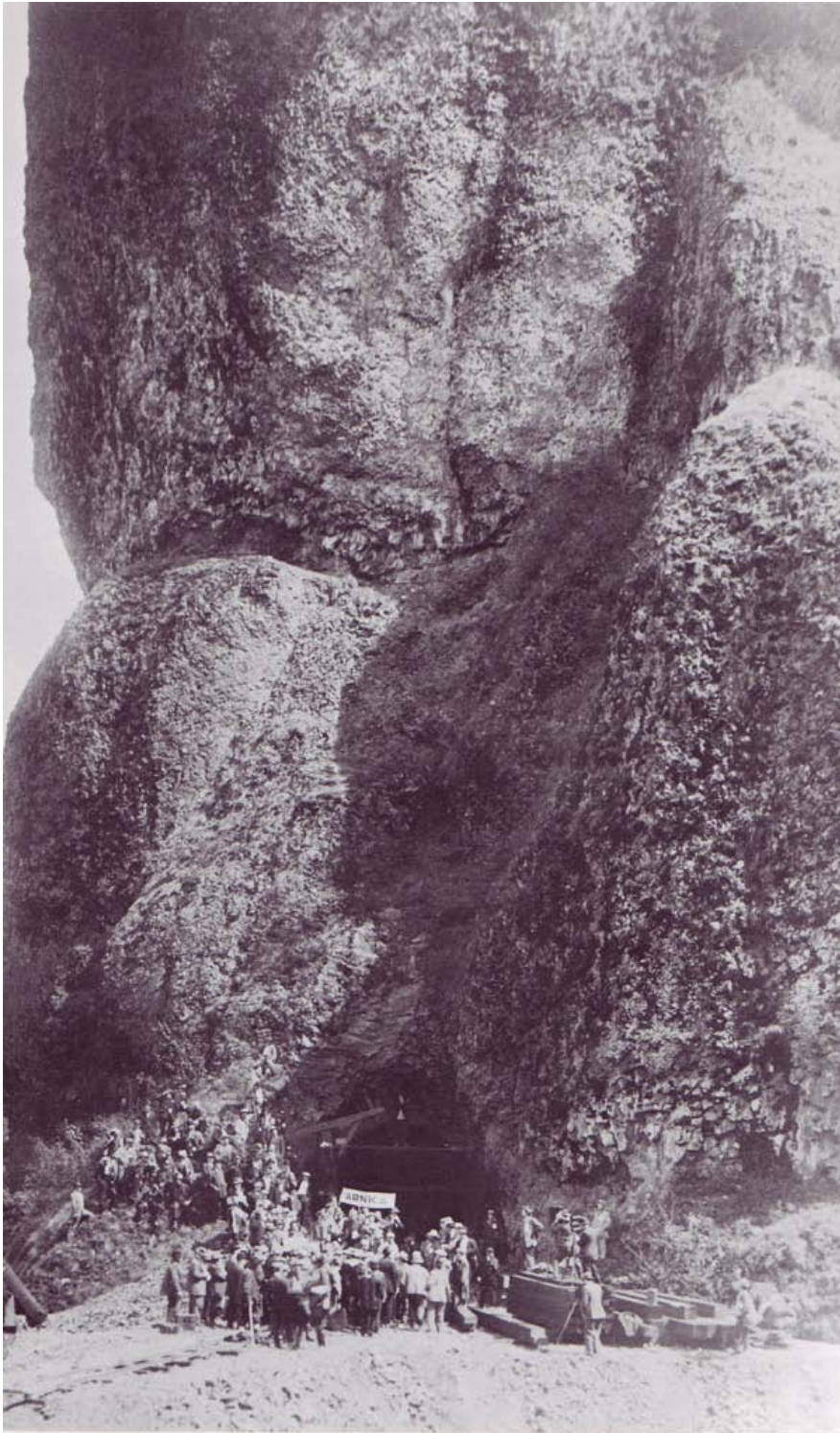
Construction of the Columbia River Highway, Oneonta Tunnel.
