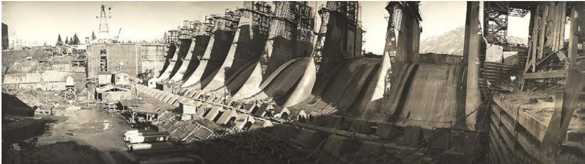
The Partially Finished Spillway.
