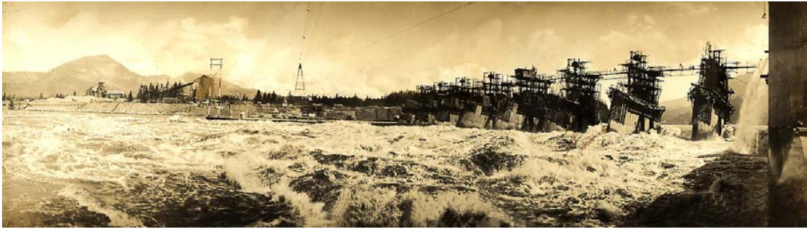
The spillway with the river flowing underneath.
