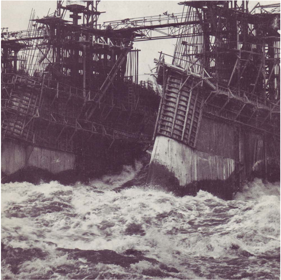
Detail of the Spillway Piers During Construction.
