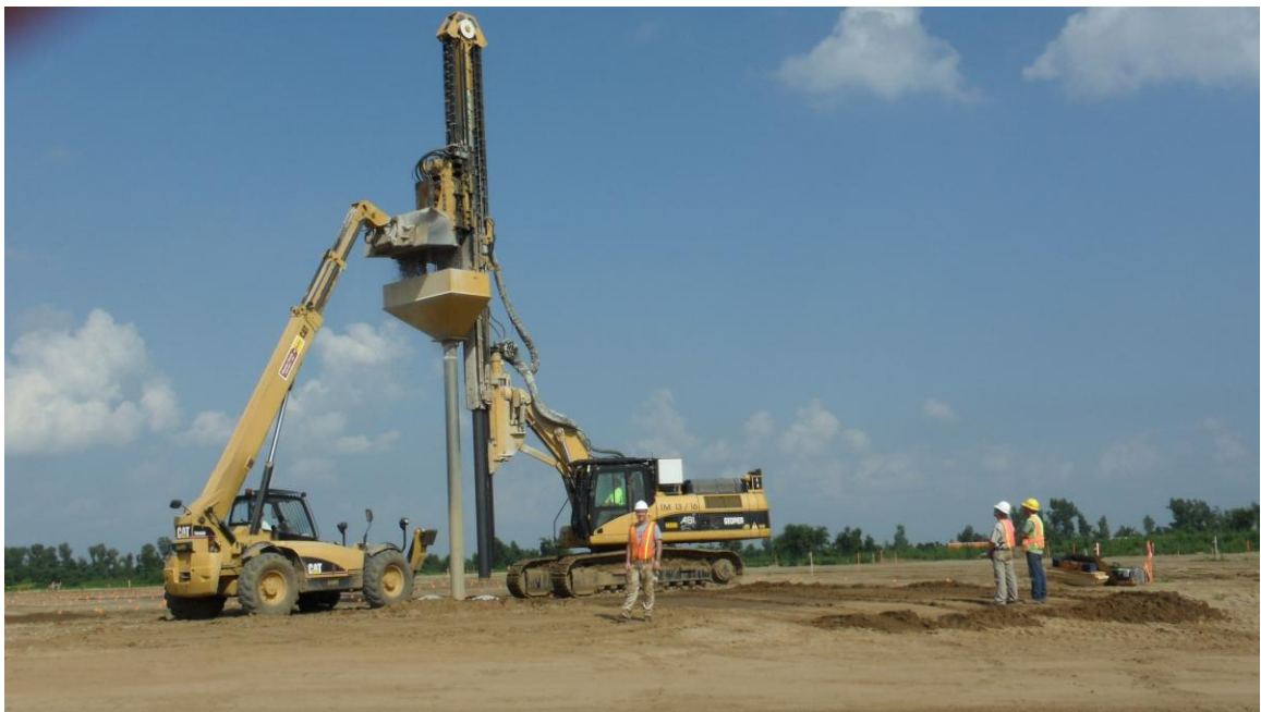
Figure 6-4. Installing an impact pier at the New Madrid, MO testing site.
