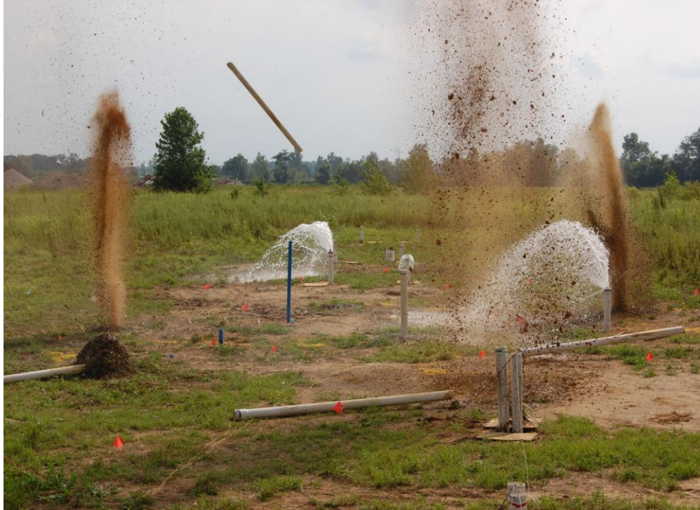
Figure 4-26. Explosive densification at Griffin, IN (photo courtesy of Roman Hryciw).
