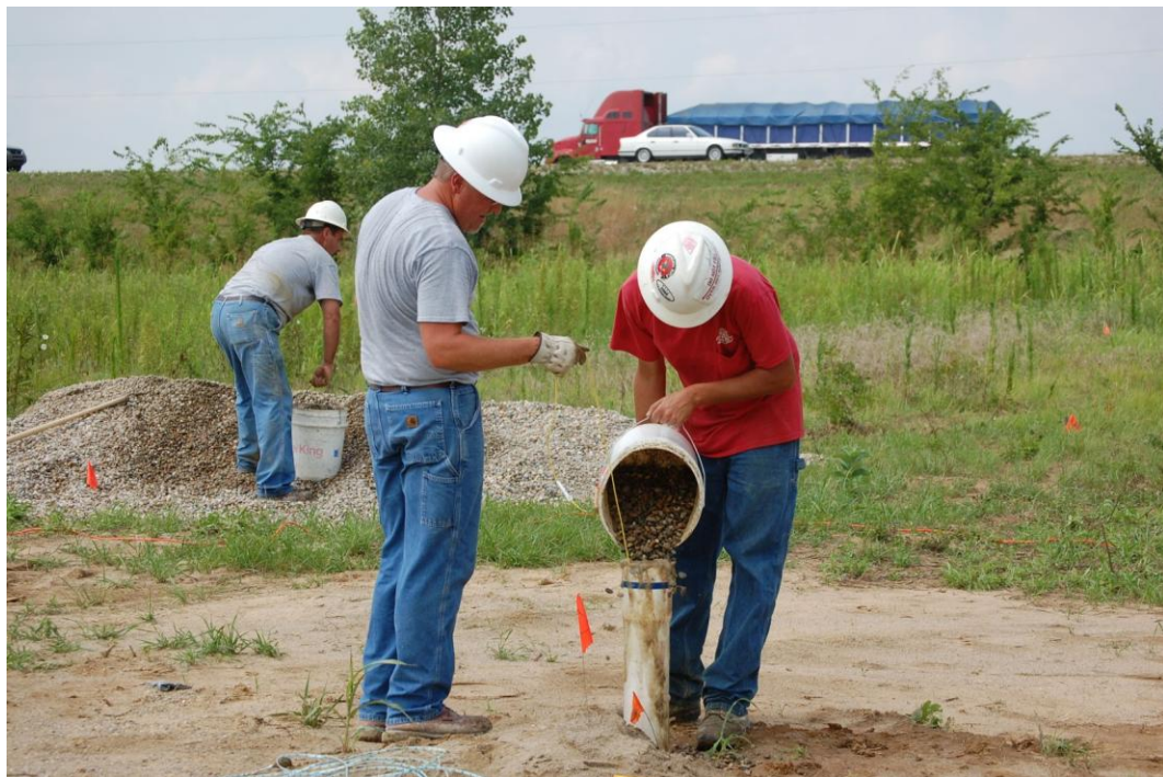
Figure 4-27. Stemming the blast hole (photo courtesy of Roman Hryciw).
