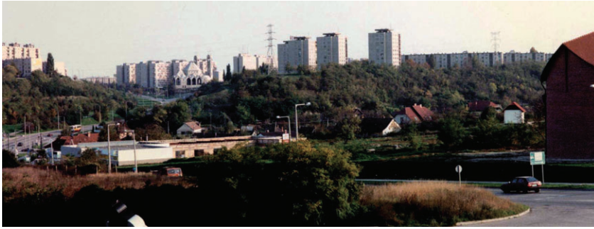
Figure 2. Dunaújváros in 1997. Panel construction apartment buildings on the plateau behind old and new family housing in the village below. Photo by author.
