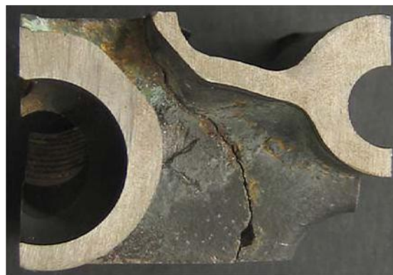
Figure 5.2.1. Crack growth in the engine head [8]
