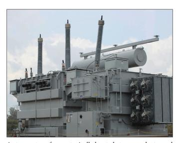
A step-up transformer typically located at power plants used to get the power out of the plant and into the transmission grid. These are potentially vulnerable assets during a GIC event and would fail en masse should a Kappenman worst-case scenario unfold. Photo courtesy of Haukur Asgeirsson.
