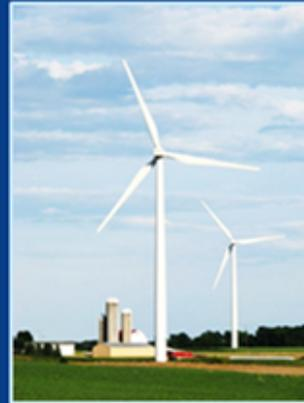
“These are the most commonly recognized form of wind turbine here in the United States, using blades (that resemble airplane propellers) to turn around a single horizontal axis. These turbines are usually exceptionally tall, in order to capture the higher velocity winds in the higher atmospheres. Horizontal axis turbines are the most commonly used turbines in today’s market, comprising almost all utility grade turbines globally.
