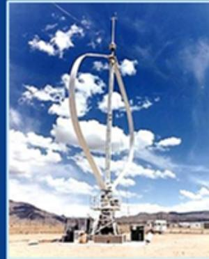
“The vertical axis variety of windmill involves two blades, rotating on a vertical axis, usually referred to as an “eggbeater” structure. The style is closer to ground than the horizontal variety, which increases the energy produced per unit construction material purchased. In addition, its vertical nature allows the structure to capture wind energy from whatever direction the wind is blowing, without the use of extra technologies.
