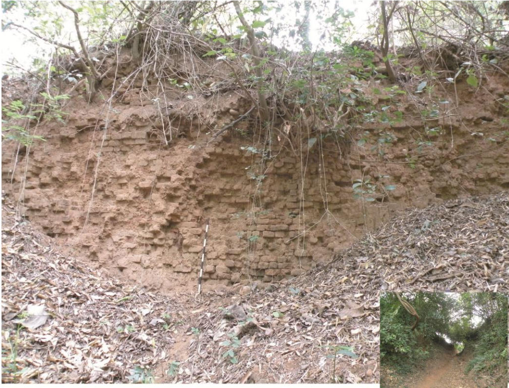
Figure 6-3: West entrance brick construction and path (inset)
