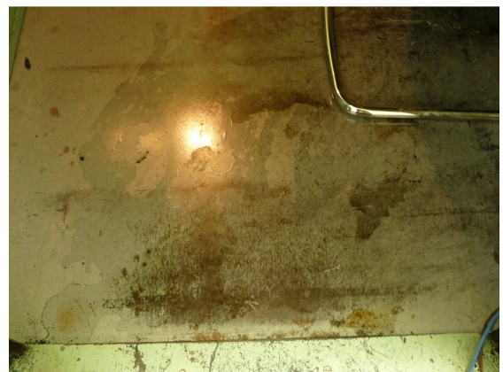
The testing room floor. Note the shiny, discolored appearance.
