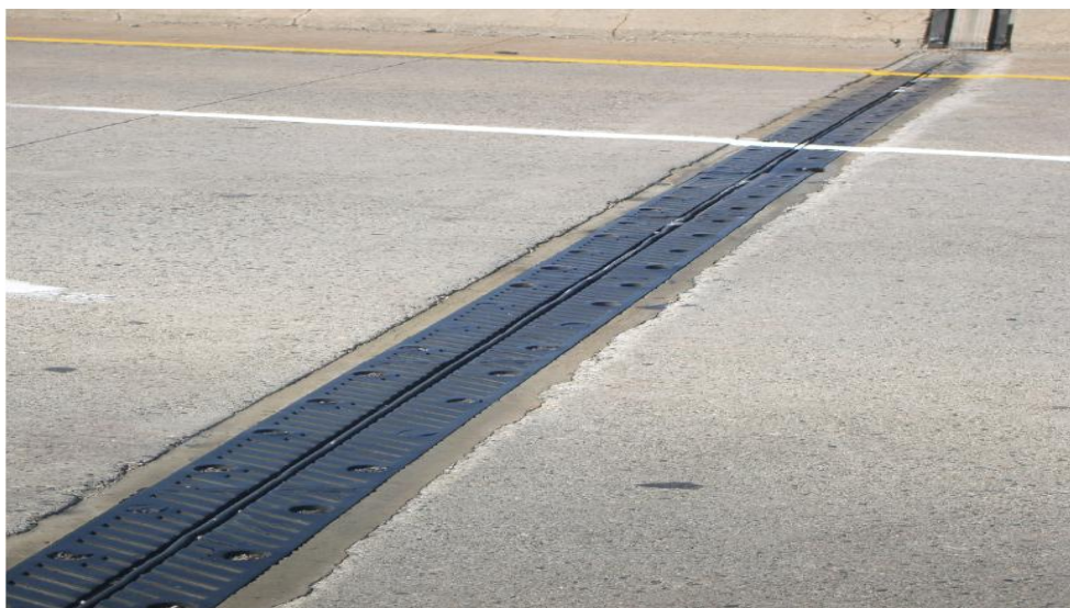
Figure 7.28: Strip seal expansion joint in the CSB
