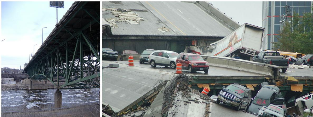
Figure: 7.3: (Left) I-35W Bridge in Minneapolis and (right) its catastrophic failure at 6:05 PM on August 01, 2007 (Image courtesy Associated Press)
