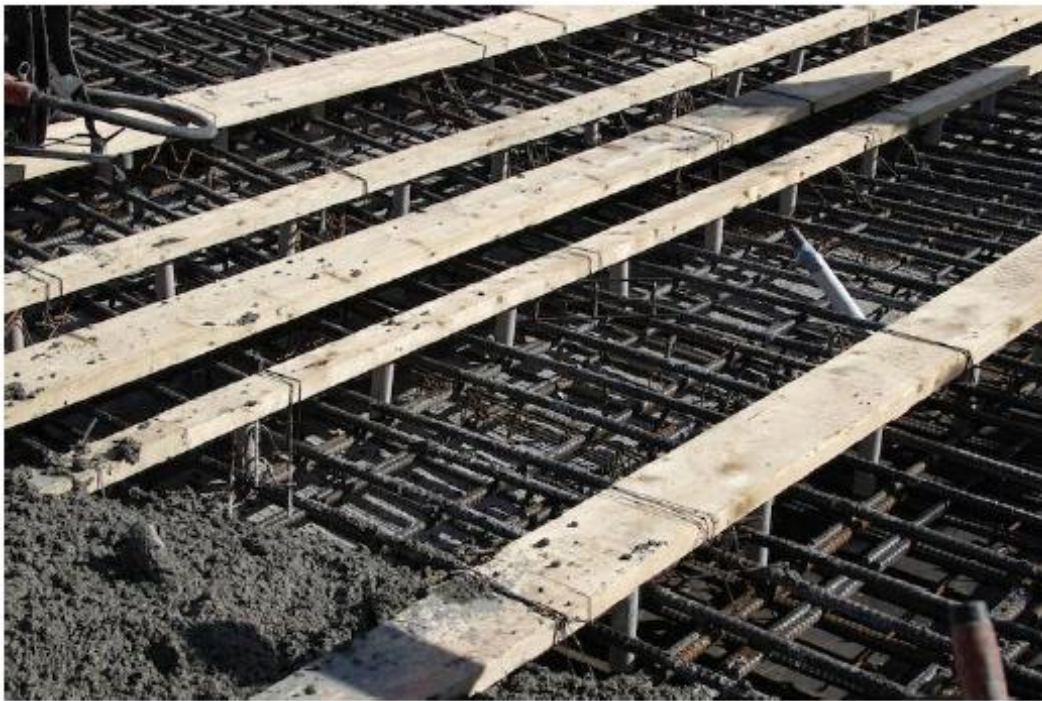
Figure 4.3: A railway bridge deck with dowels and wooden planks installed
