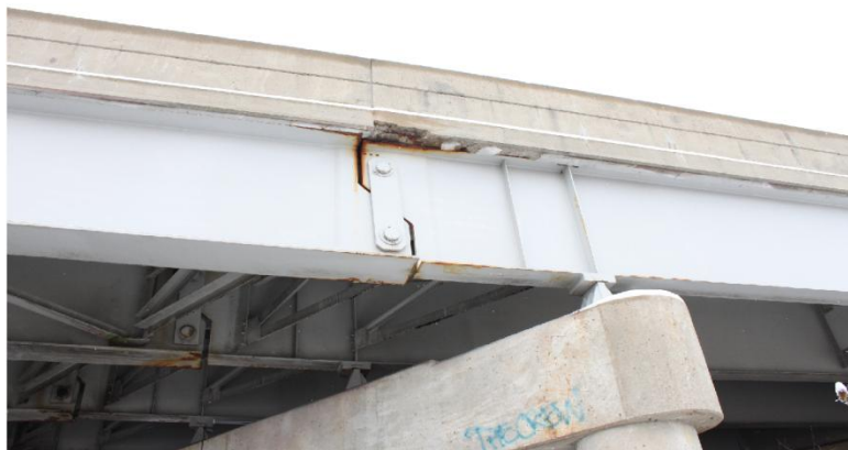
Figure 7.23: Pin and hanger assembly in the CSB
